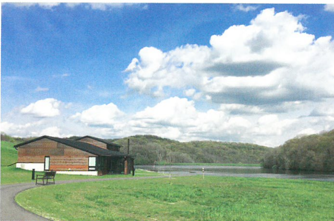
05.16.19 The ADA path curves towards the building and extends access down to the lake.
