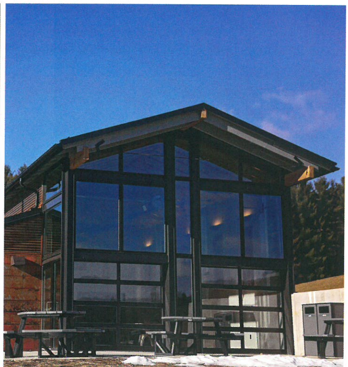
01.08.19 Glass garage doors open the community room onto Prairie Smoke Terrace.
