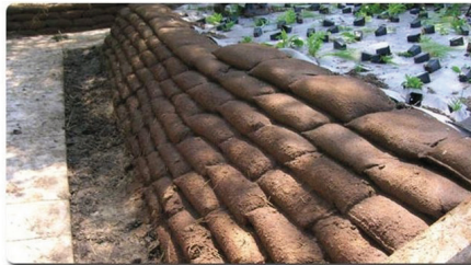
Day 1. Soil-filled geotextile bags are hydro-seeded or planted with native plant plugs.
