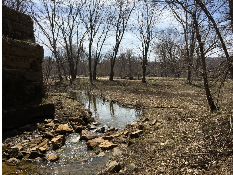
Photograph 7 Down stream looking towards the Baraboo River
