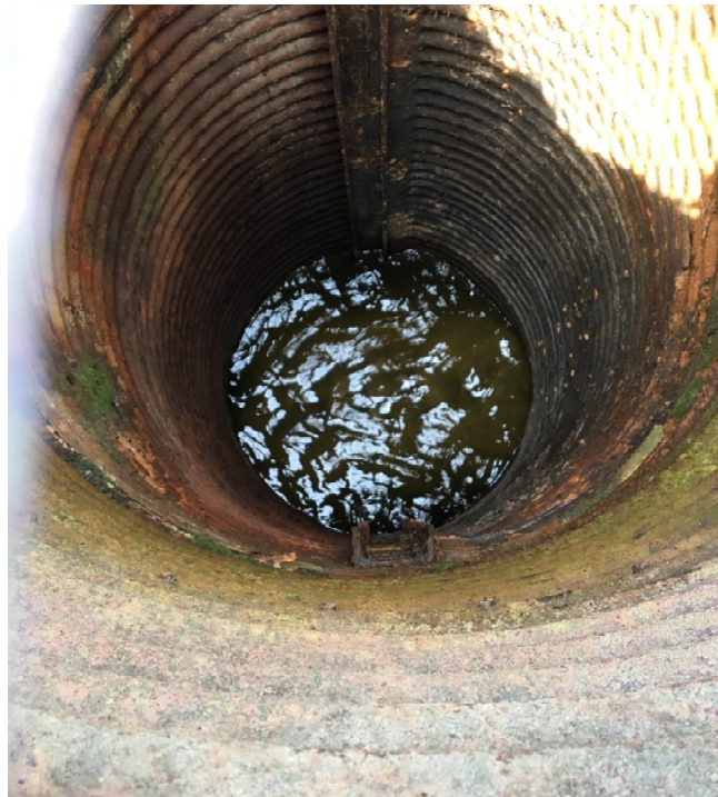
Photograph 6 Drop Inlet Structure
