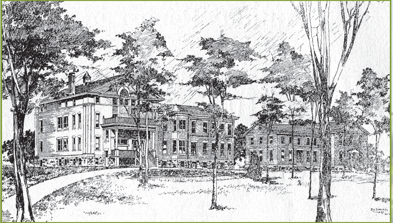
Drawing of the original buildings at the County Farm circa 1895. Photo courtesy of the Sauk County Historical Society.
