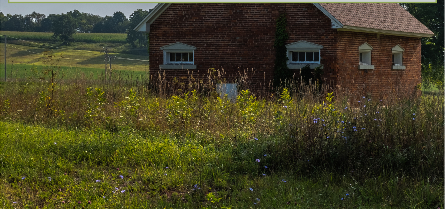
View of the back of fire house. Photo courtesy of Maxwell Lohse.
