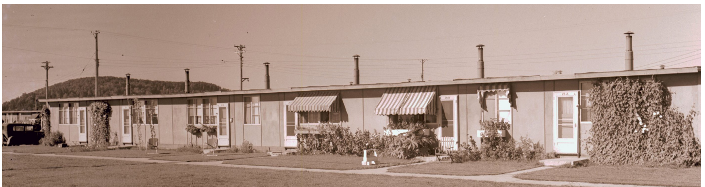
Six Unit Apartment Building, World War II Era (Courtesy of Badger History Group)
