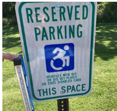
Low-Level Deficiency Raise signage to proper height.
