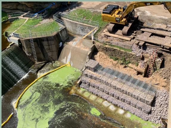
After many months working with the surrounding land owners and WI DNR the Delton Dam project has finally started. Staff have been on site almost daily to keep an eye on the water levels. Along with attending weekly project meetings. Improvements include installation of Erosion control measures and a turbidity barrier, demolition has started on the concrete overlook area, and excavation of the area for the gabion baskets (pictured).
