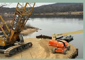
Staff attended a preconstruction meeting with MSA Professional Services and Zenith Tech, the prime contractor for the project. An access road to the job site where the crane has been stationed has been installed along Water Street. The job site will provide access to the existing bridge as well. Pilings were installed to extend their platform base for the crane and other equipment.
