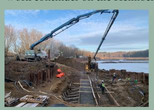
The concrete work is 100% completed, and Janke General Contractors is awaiting on the stop logs to be constructed. The last rainfall set us back, as the soil to be used for back filling is predominantly clay. The soil originally met the compaction test prior to the rain, but has since failed. The soil will need to dry out before Janke is able to back fill.
