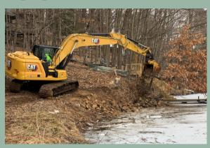
Riprap was installed along the beach shoreline at Lake Redstone County Park. The shoreline, along with the neighboring property's 10' of shoreline, was experiencing erosion. The Highway Department assisted in the project, using a track skid steer to haul riprap down to the beach and an excavator to place it.
