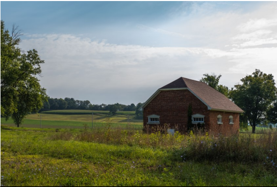
Historic fire house building. Photo courtesy of Maxwell Lohse.
