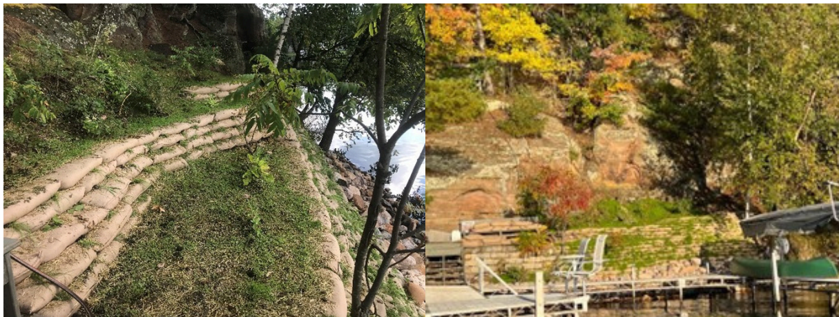
Completed Installation of Geotextile Bags with Riprap on Lake Redstone
