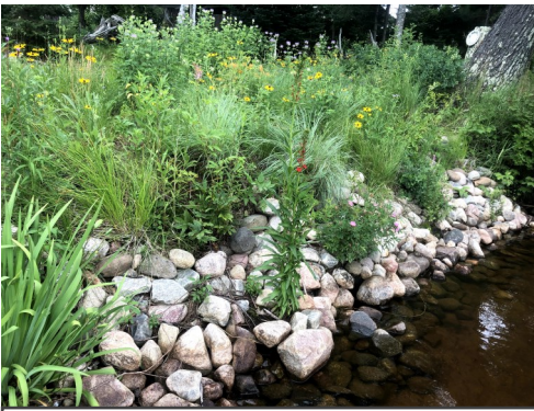
Example of vegetated rock riprap along shoreline of lake.
