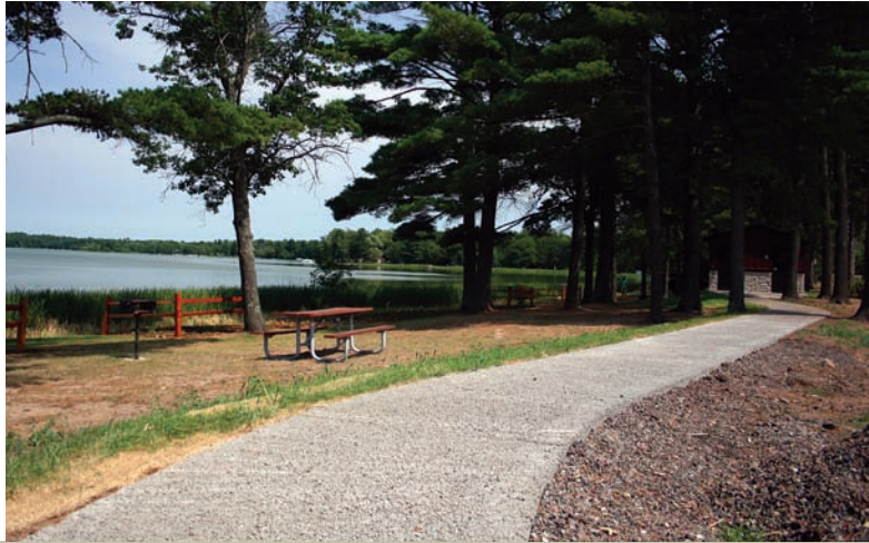
Porous concrete sidewalk at the Clam Narrows boat landing in Burnett County.
