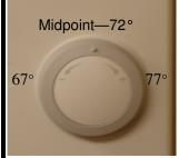
Thermostats, especially in the hallways and common areas, should be left in the mid point—straight up position—to help ensure a constant, comfortable temperature. Adjusting the thermostat is a temporary thing. If you need the temperature adjusted higher or lower, maintenance can adjust it from the computer to a more comfortable temperature. Resident rooms should be set at the most comfortable position for that resident and should be adjusted only at the resident's request.
