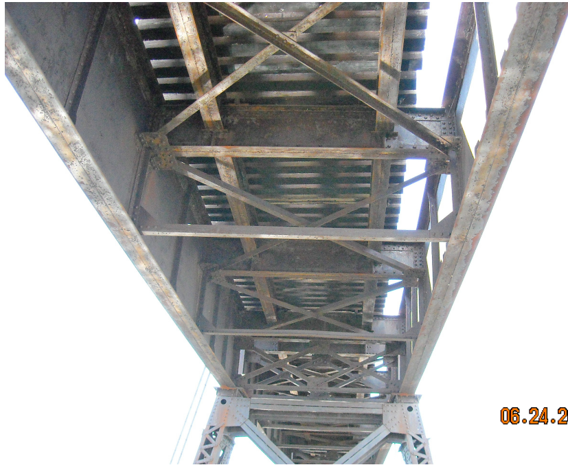
Figure 2-2 Typical View of Deck Girder System
