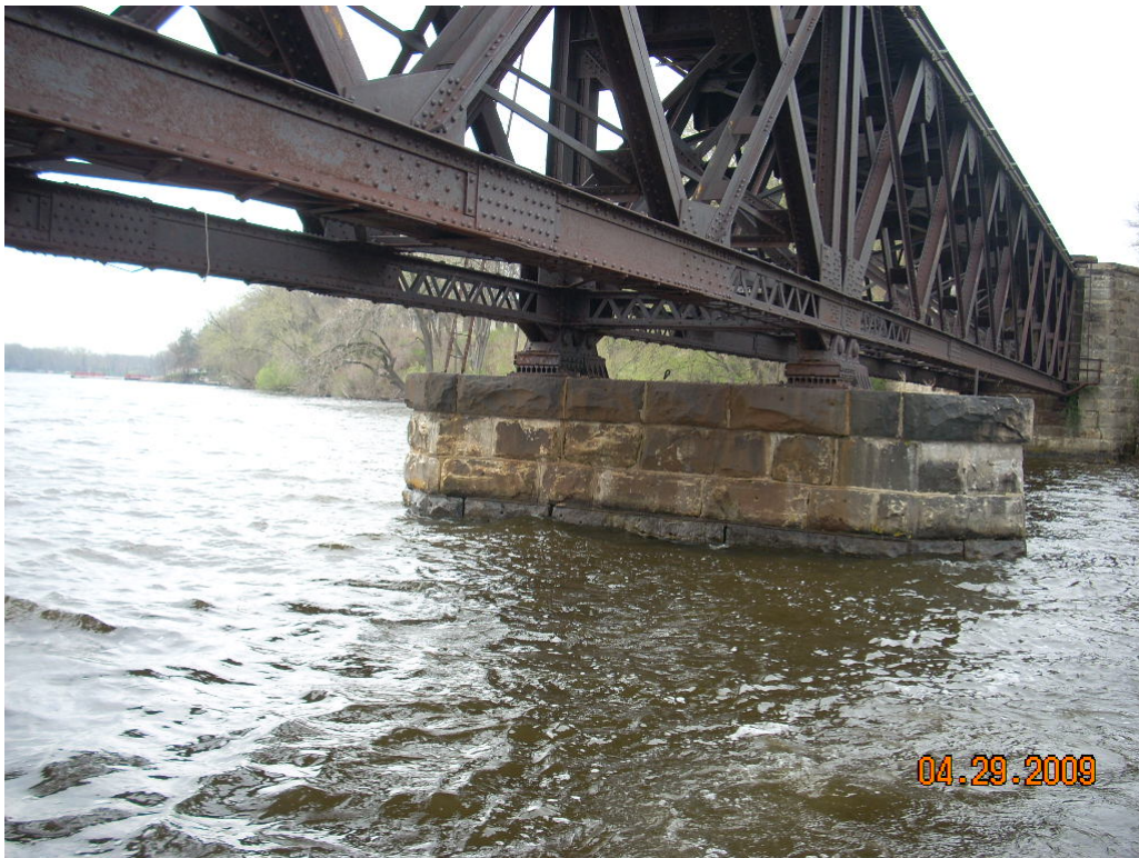
East Side of Pier 22
