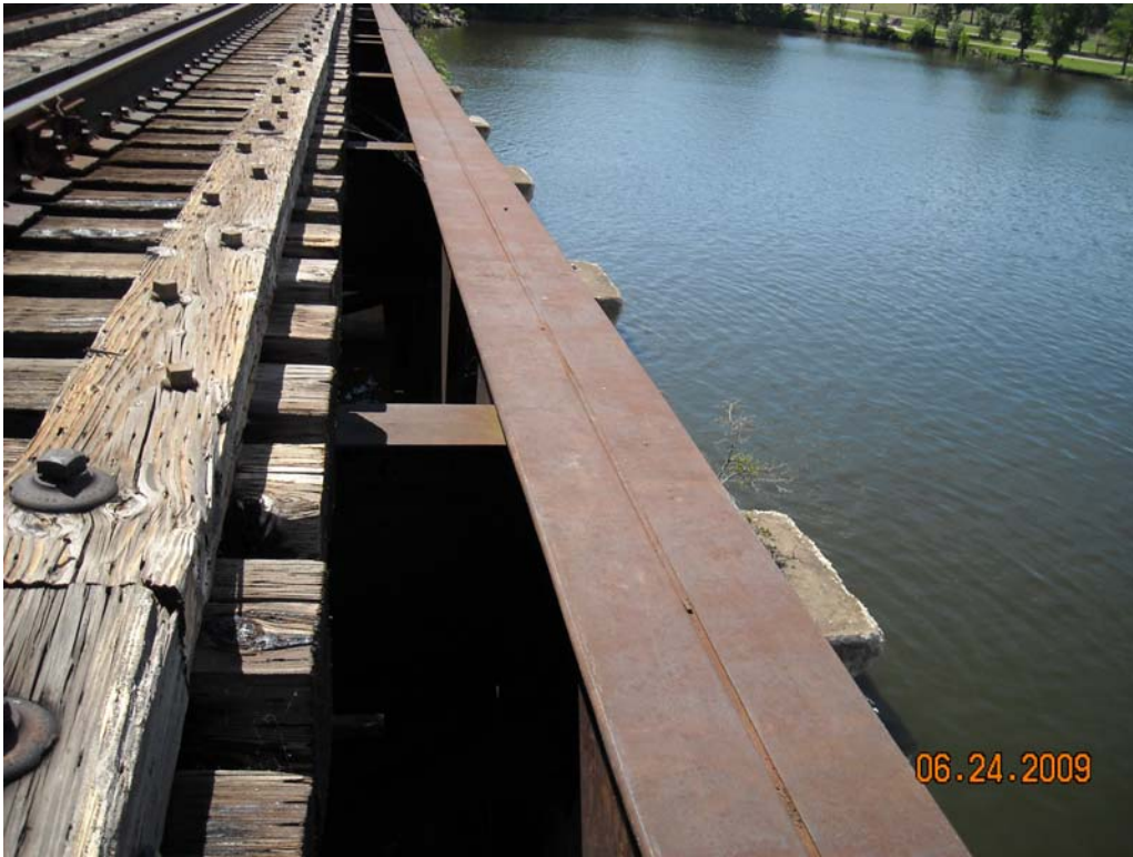
Typical Top Flange of Deck Girder
