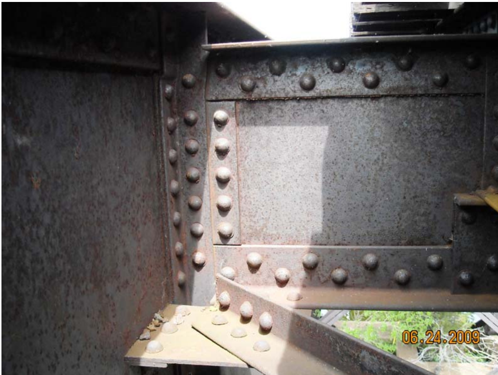
Typical Top Side of Floor Beam to Deck Girder Connection
