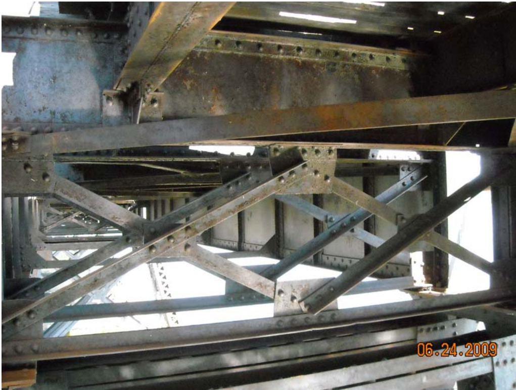
Typical Floor Beam and Cross Frame at Pier
