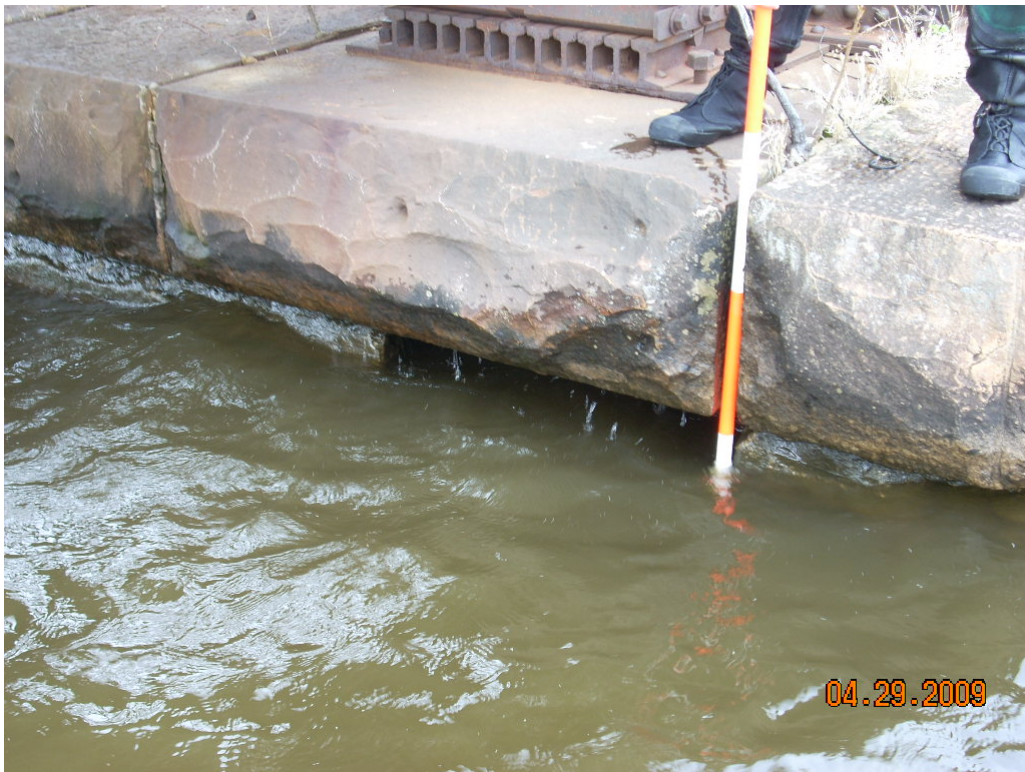
Pier 2 at south (DS) bearing has a missing block on the west face at the waterline
