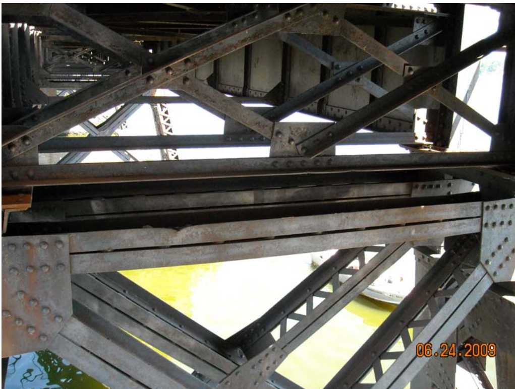
Typical Cross Frame and Top of Steel Tower at Pier
