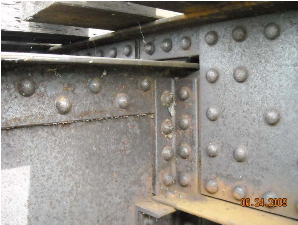
Typical Stringer to Floor Beam Connection
