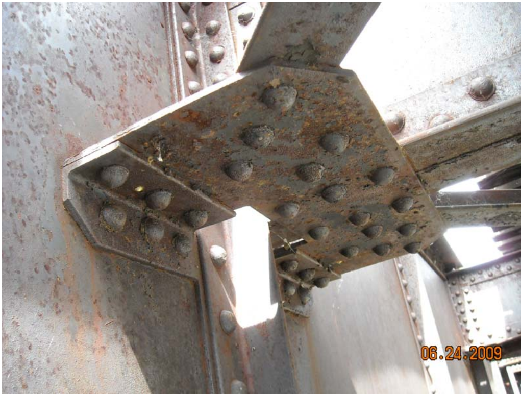
Typical Bottom Side of Floor Beam to Deck Girder Connection
