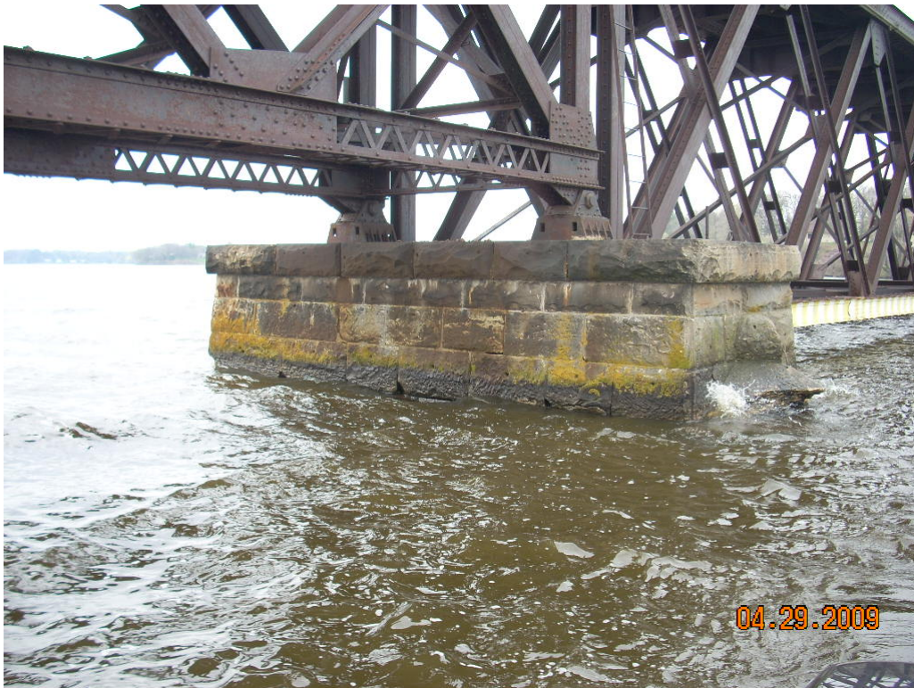
East Side of Pier 18
