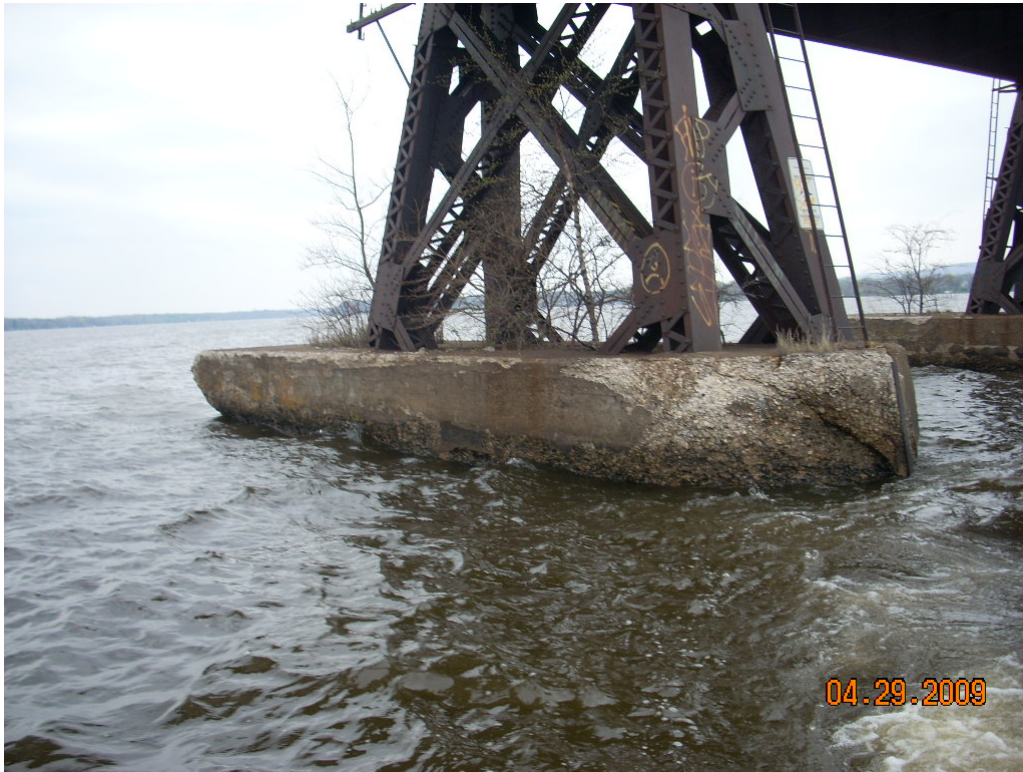
East Side of Pier 5
