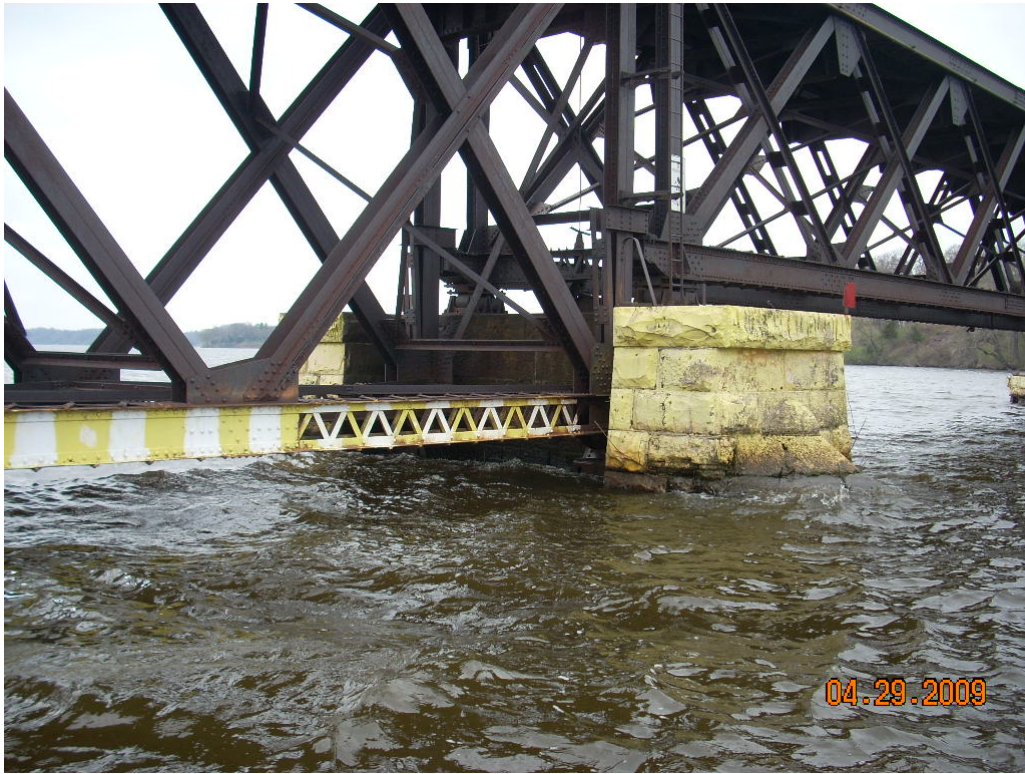
East Side of Pier 19
