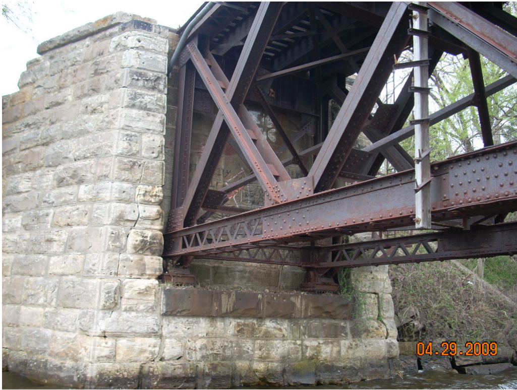
East Side of Abutment 23 (West)
