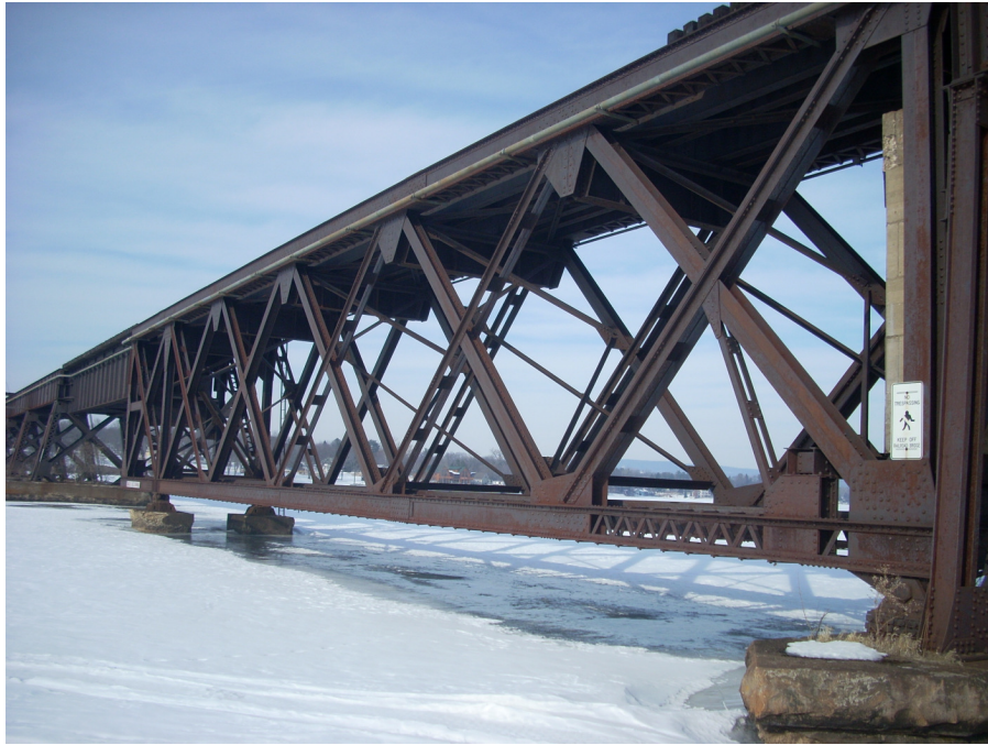
Figure 2-3 Typical View of Deck Truss System
