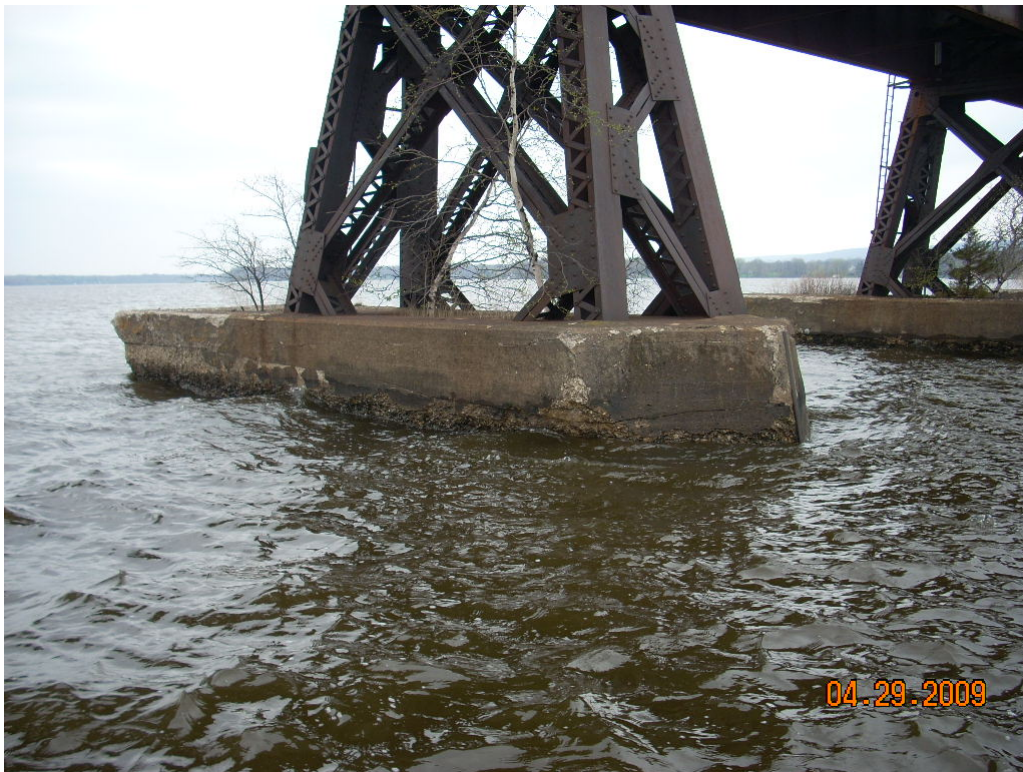
East Side of Pier 6
