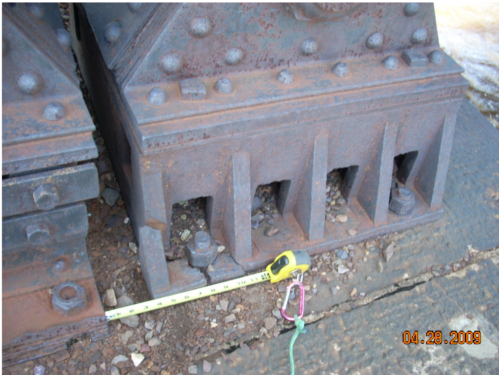
Span U NE bearing at Pier 22 has a cracked bottom plate at NE bolt.
