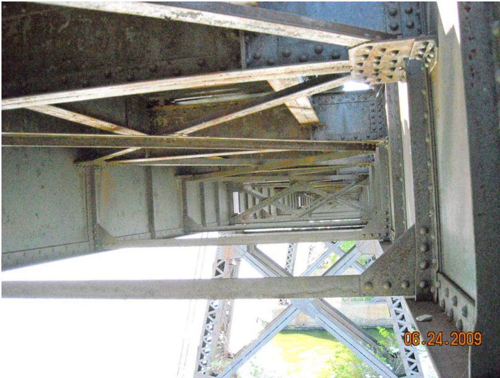
Typical Transverse and Diagonal Lateral Bracing
