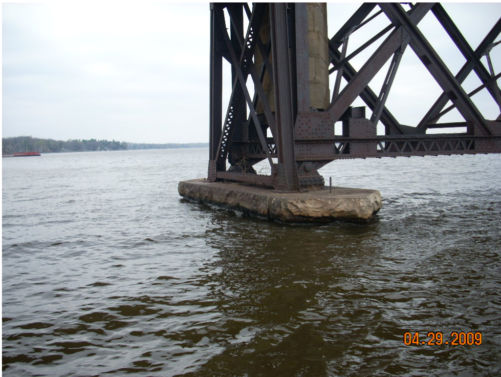
East Side of Pier 2
