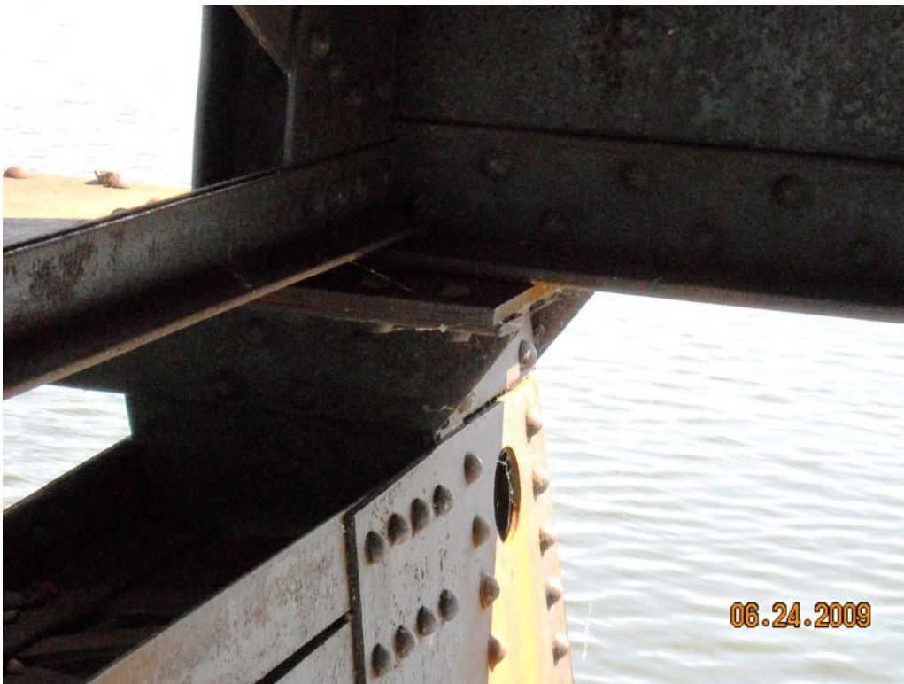
Typical Interior of Bearing
