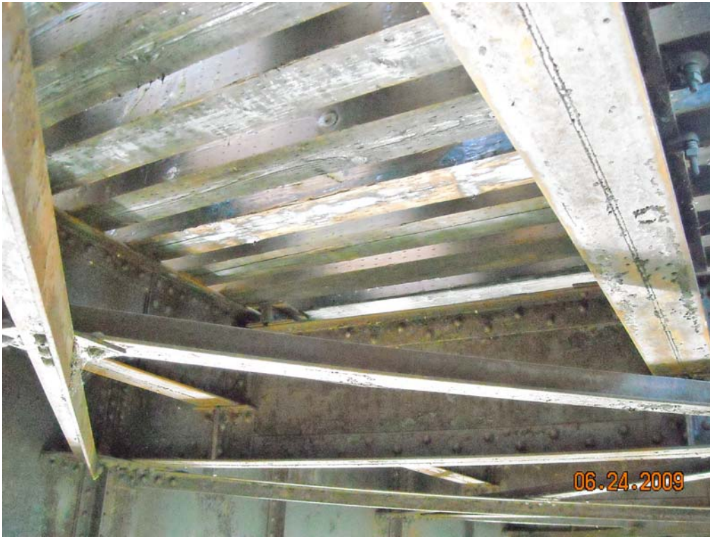
Typical Deck Underside
