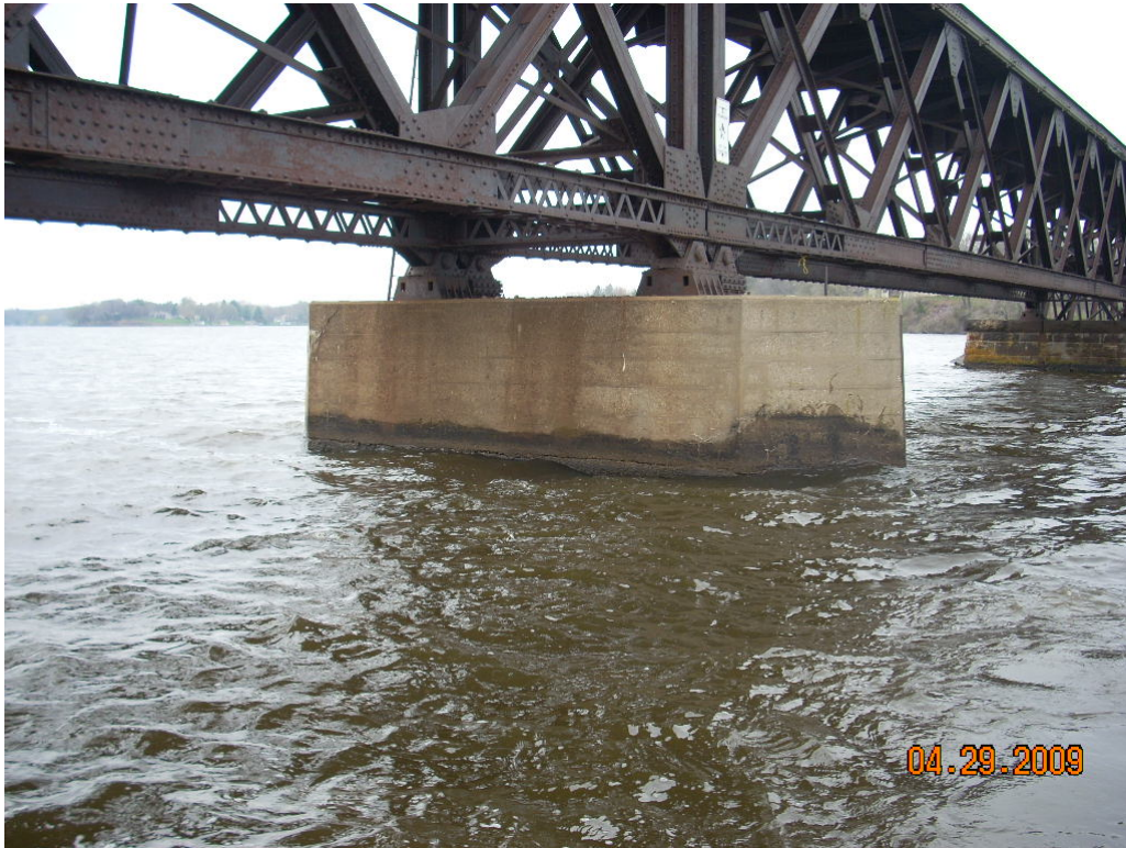
East Side of Pier 17
