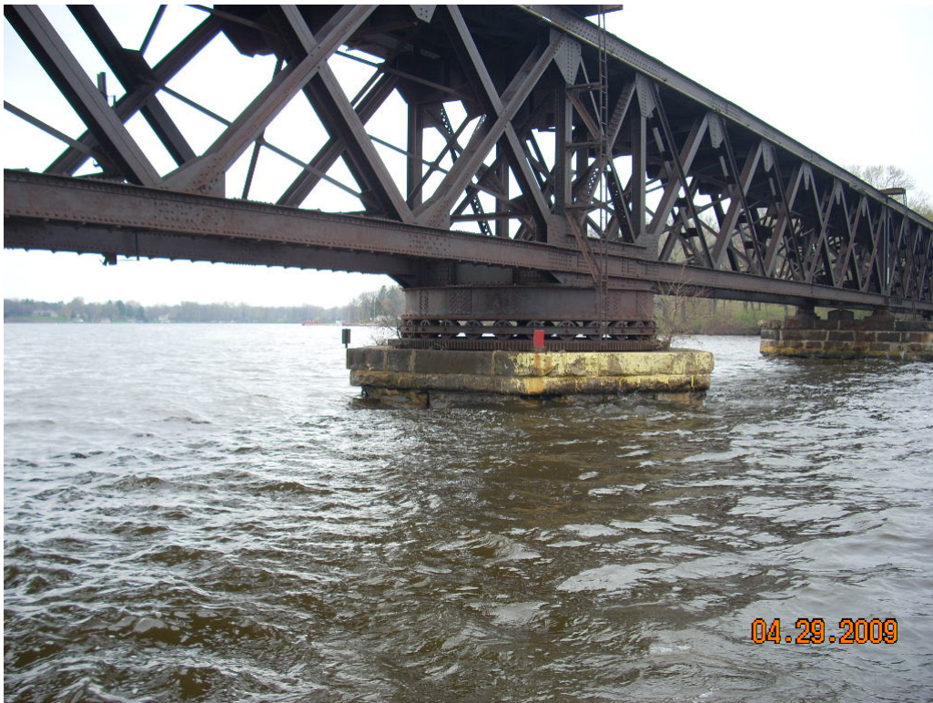
East Side of Pier 20
