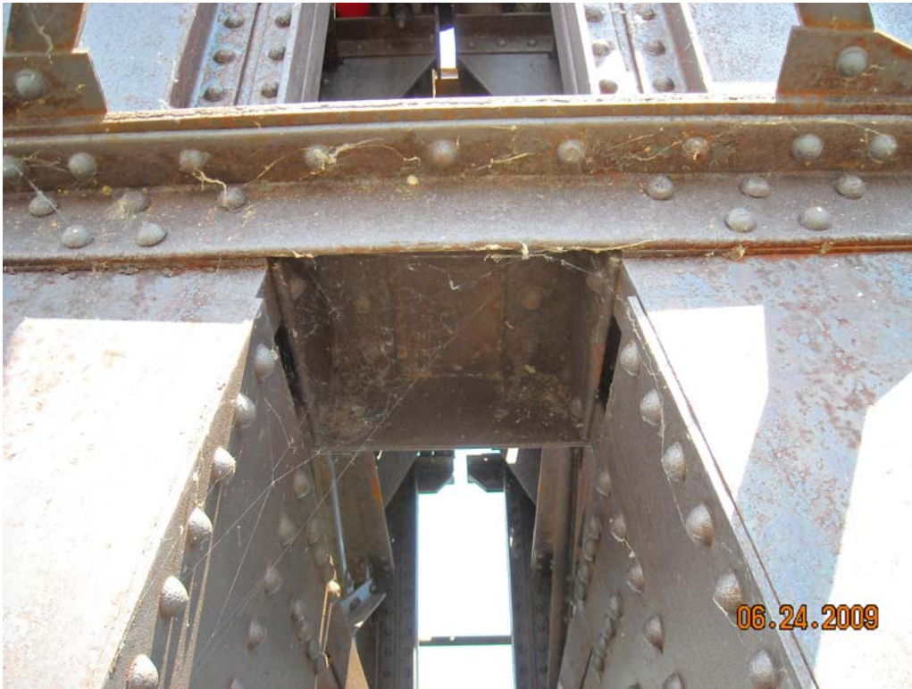
Typical Underside of Bearing Pedestal at Top of Steel Tower
