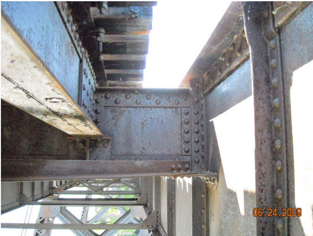
Typical Stringer to Floor Beam and Floor Beam to Deck Girder Connections
