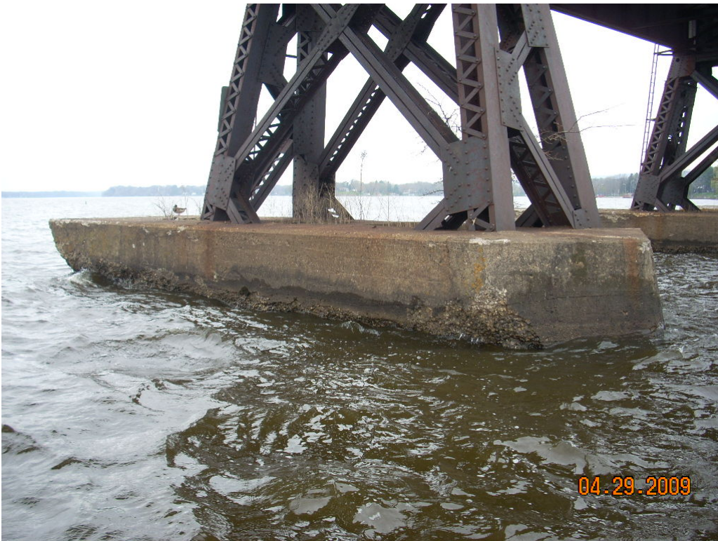
East Side of Pier 12
