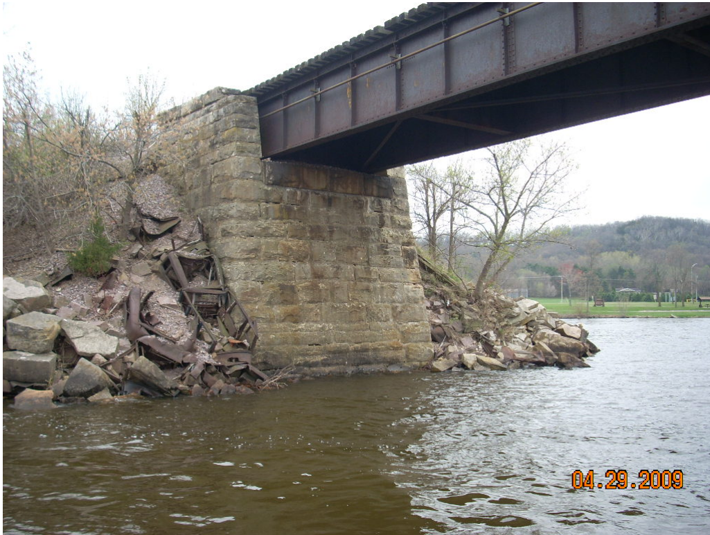
West side of Abutment 1 (East)
