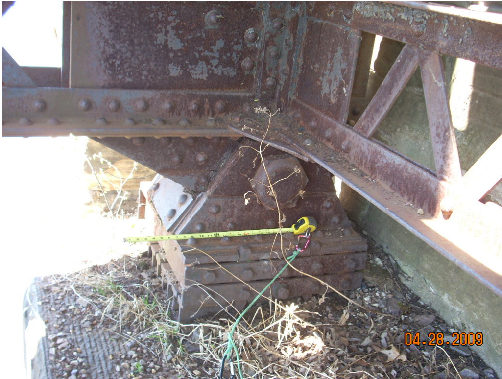
Typical bearing at Abutment 23 (West)
