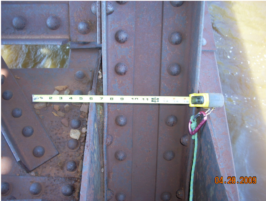
Typical pack rust up to 5/8 inch between diagonal and vertical gusset plate at lower chord
