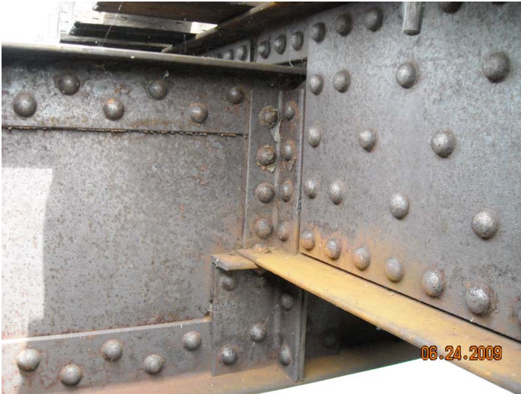
Typical Stringer to Floor Beam Connection
