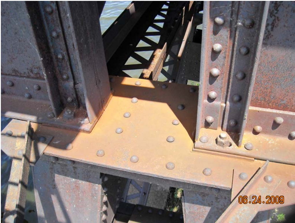
Typical Exterior of Bearings
