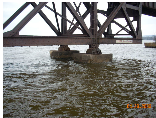
Figure 7-5 Span B Truss.
