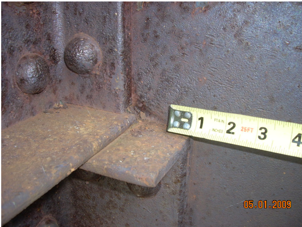
Typical pitting up to ¼ inch deep and 1 inch tall by 3 inches wide in FB web at stringer shelf plate in Spans D through M
