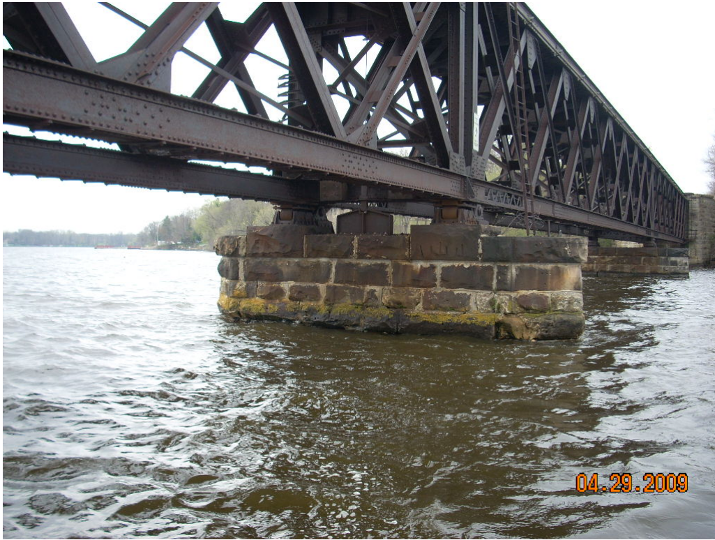
East Side of Pier 21
