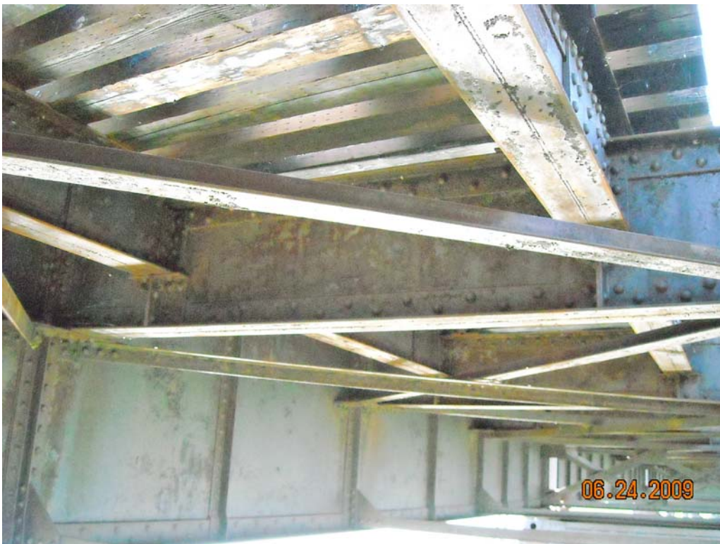
Typical Diagonal Lateral Bracing
