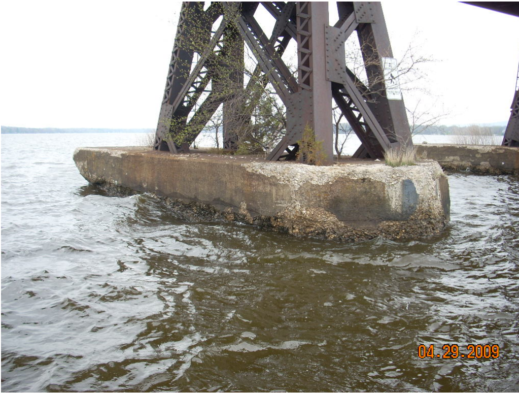
East Side of Pier 7
