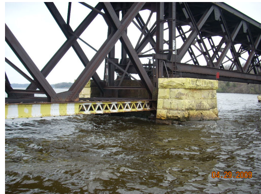
Figure 7-3 Pier 19 Bearings.
