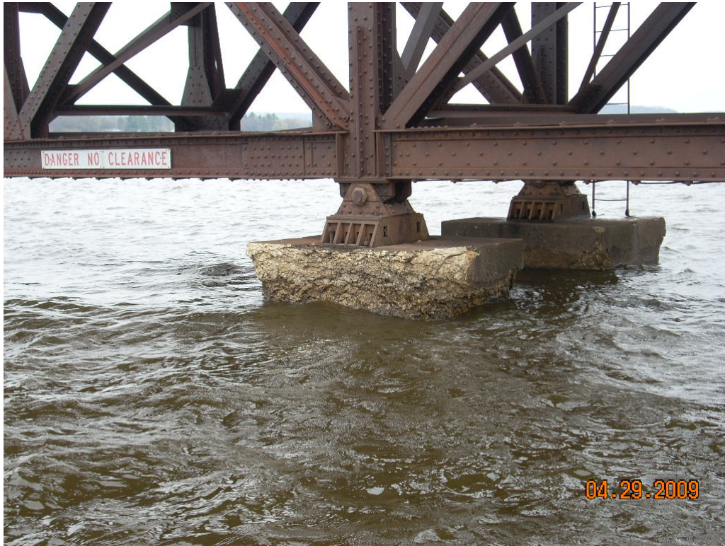
Pier 3 south (DS) bearing pedestal has spalling with exposed steel at the SE corner
