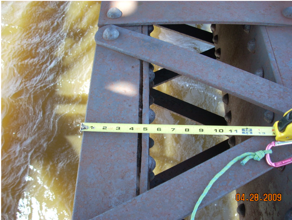
Span S North Lower Chord in 4 th bay west of Pier 20 has pack rust up to ¼ inch between the south top flange and south web plate
