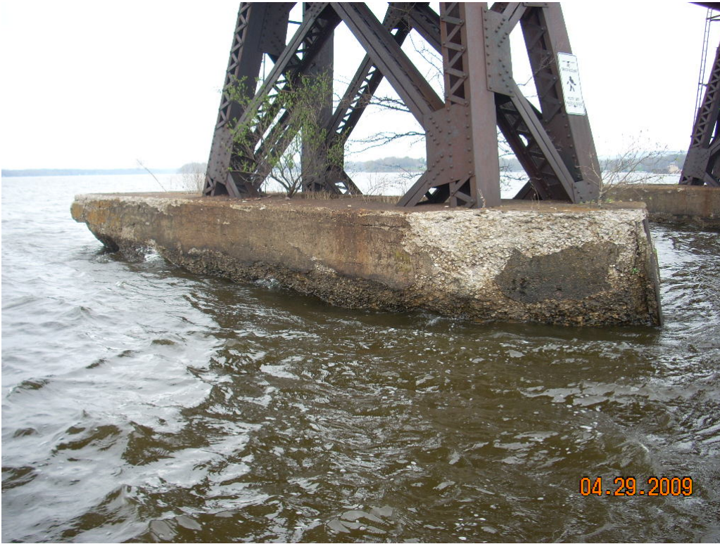
East Side of Pier 11
