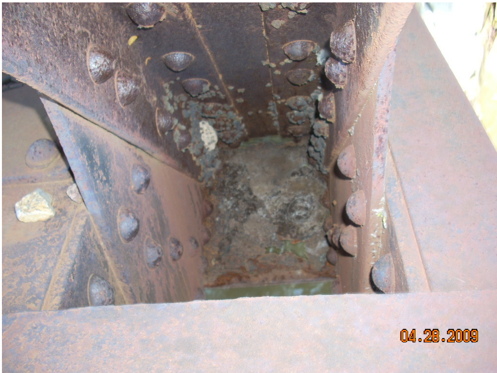
Span U batten plate at L7 on bottom of North Lower Chord has a hole
