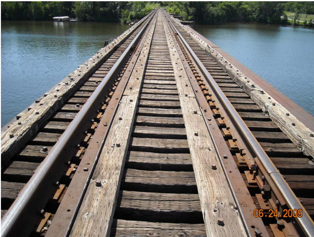
Typical Top of Deck
