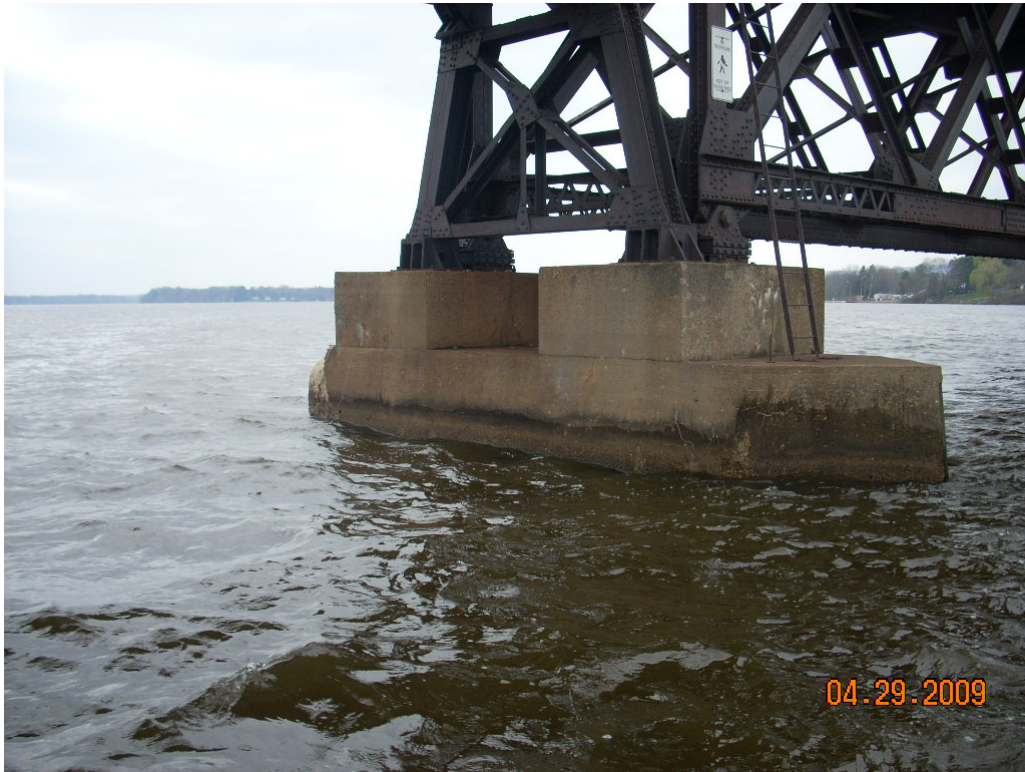
East Side of Pier 15
