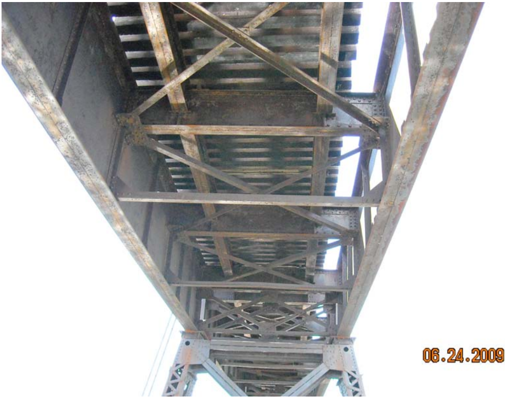
Typical Deck Girder Span
