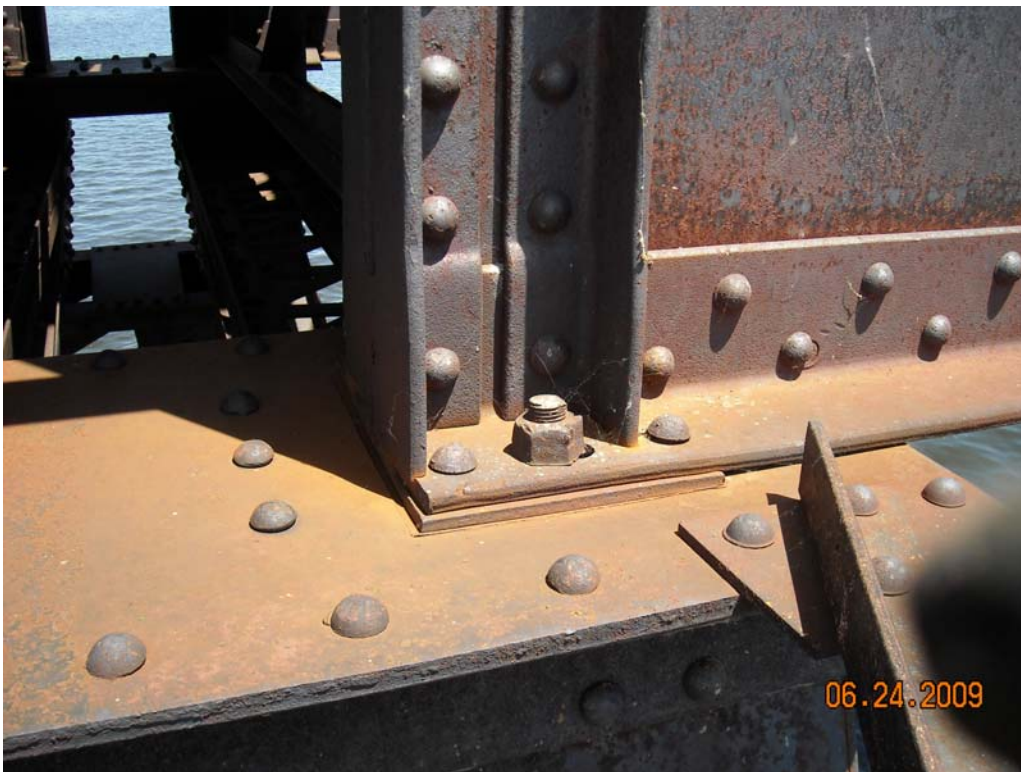
Typical Exterior of Bearing
