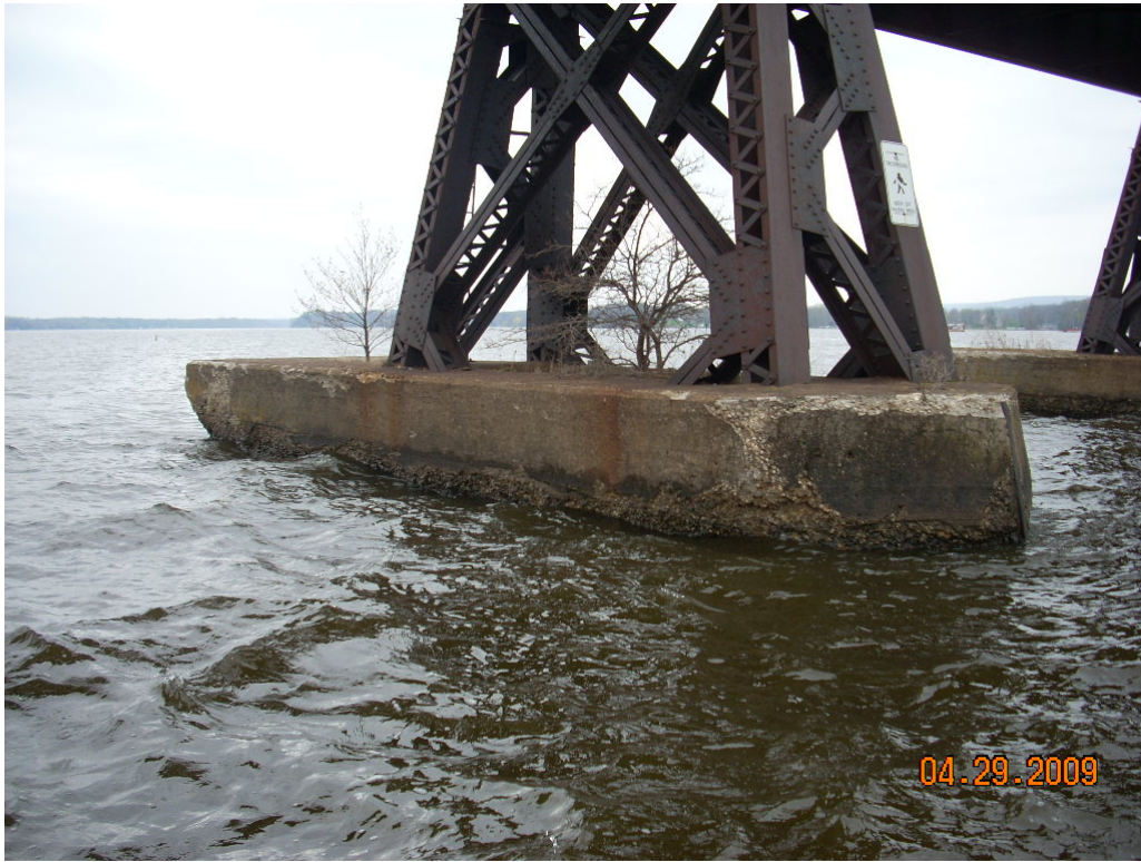
East Side of Pier 13
