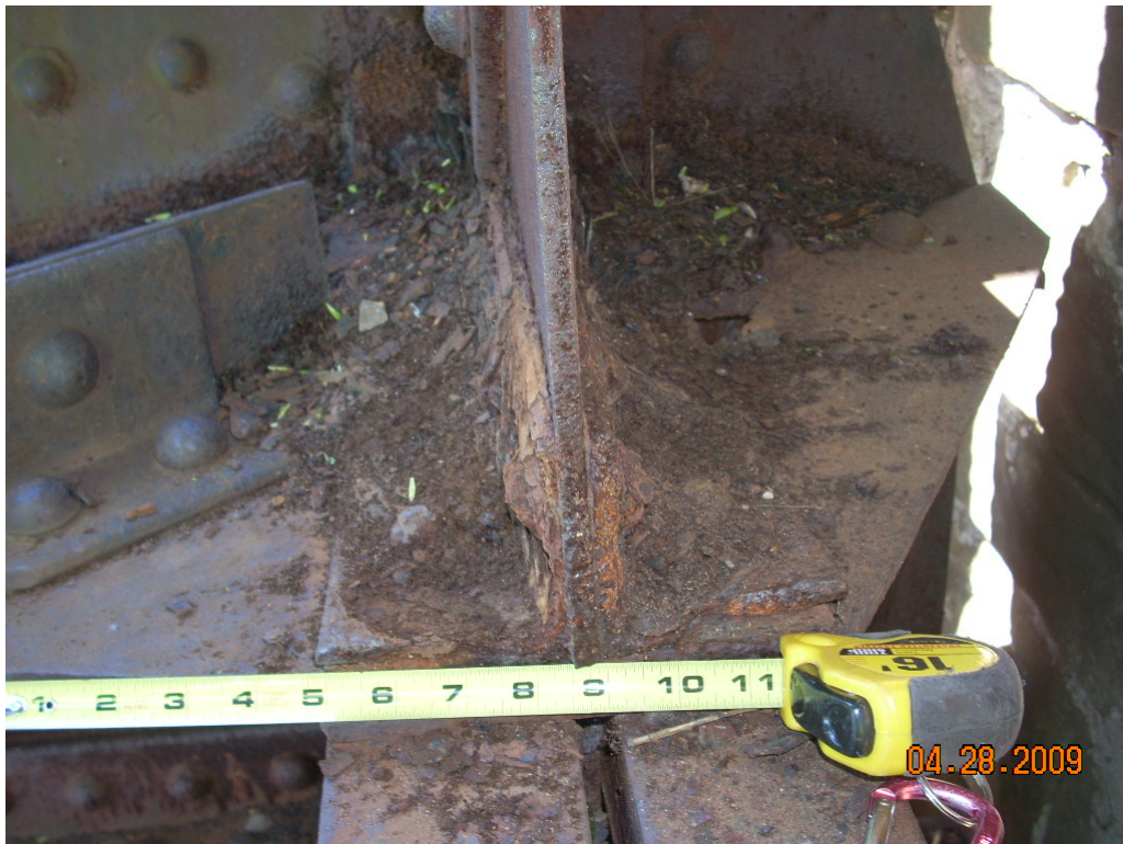
Abutment 23 has up to 50% section loss of angles on horizontal gusset plate above SW Bearing
