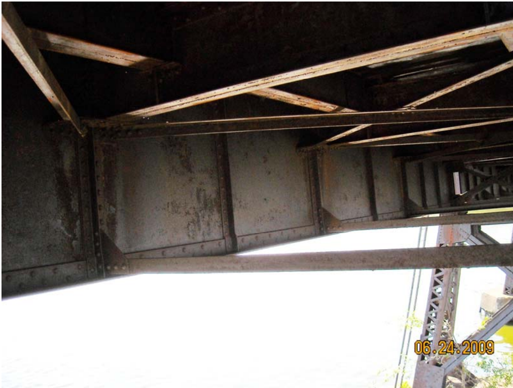
Typical Interior of Deck Girder
