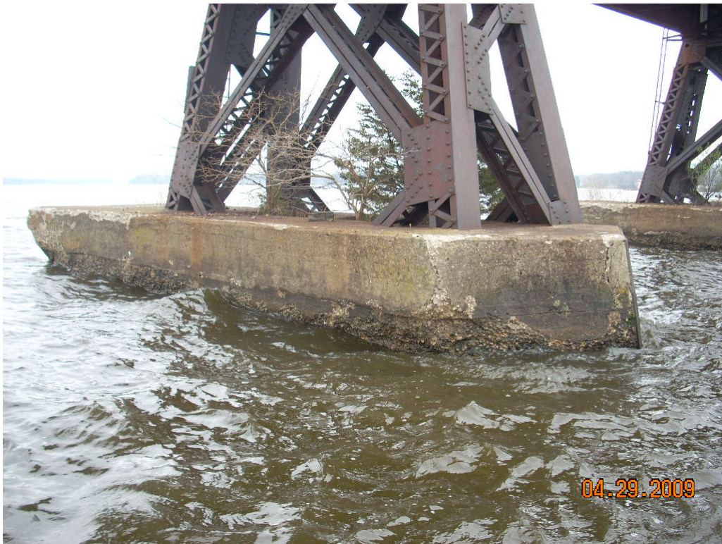
East Side of Pier 10
