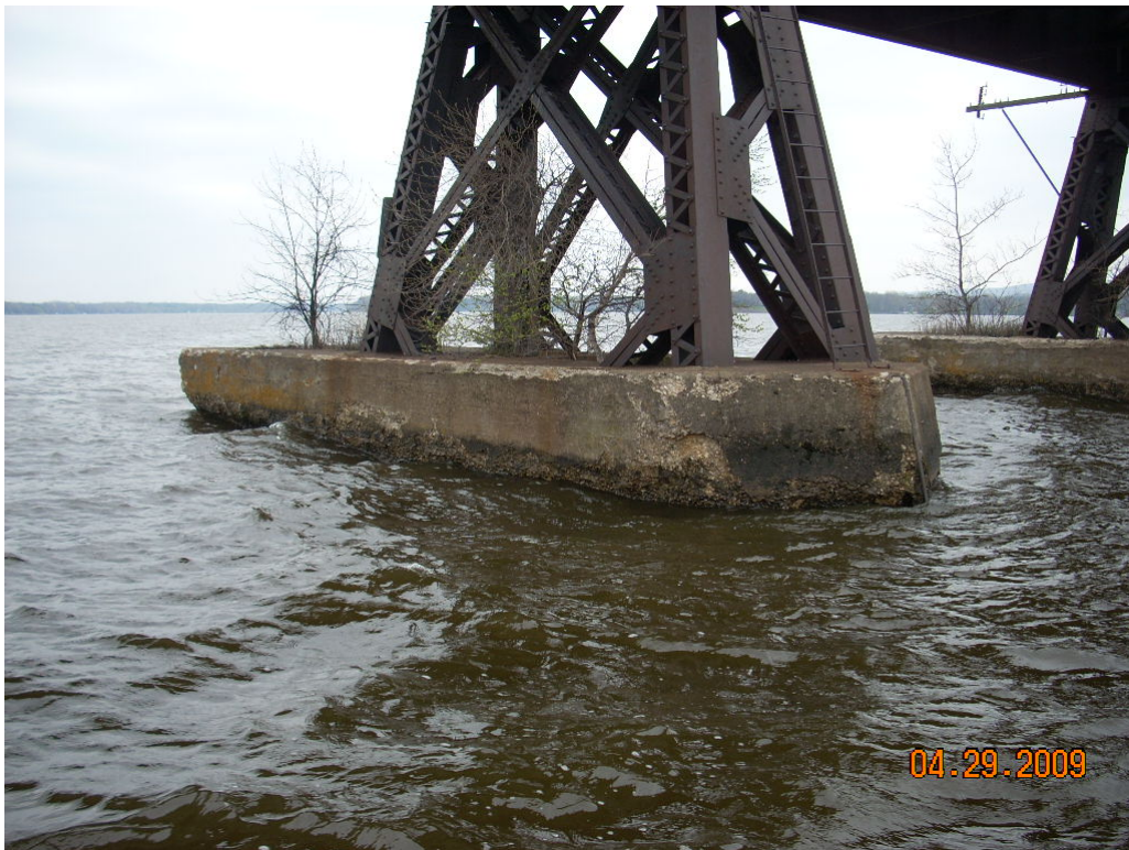
East Side of Pier 4
