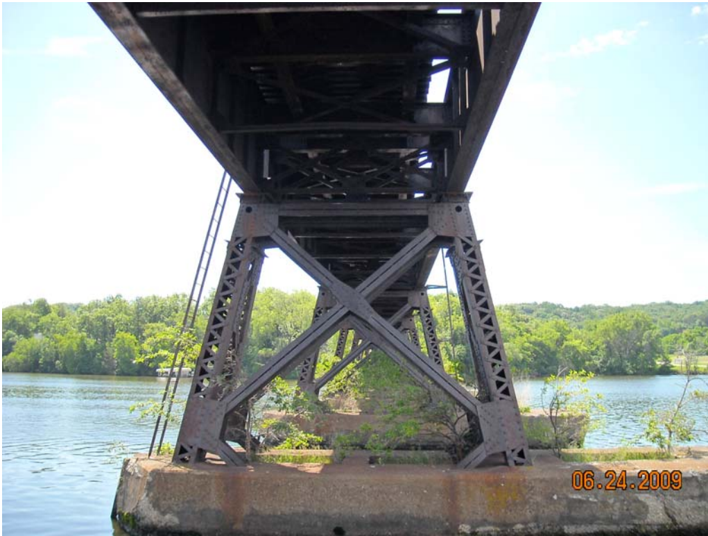
Typical Concrete Encased Steel Tower Pier
