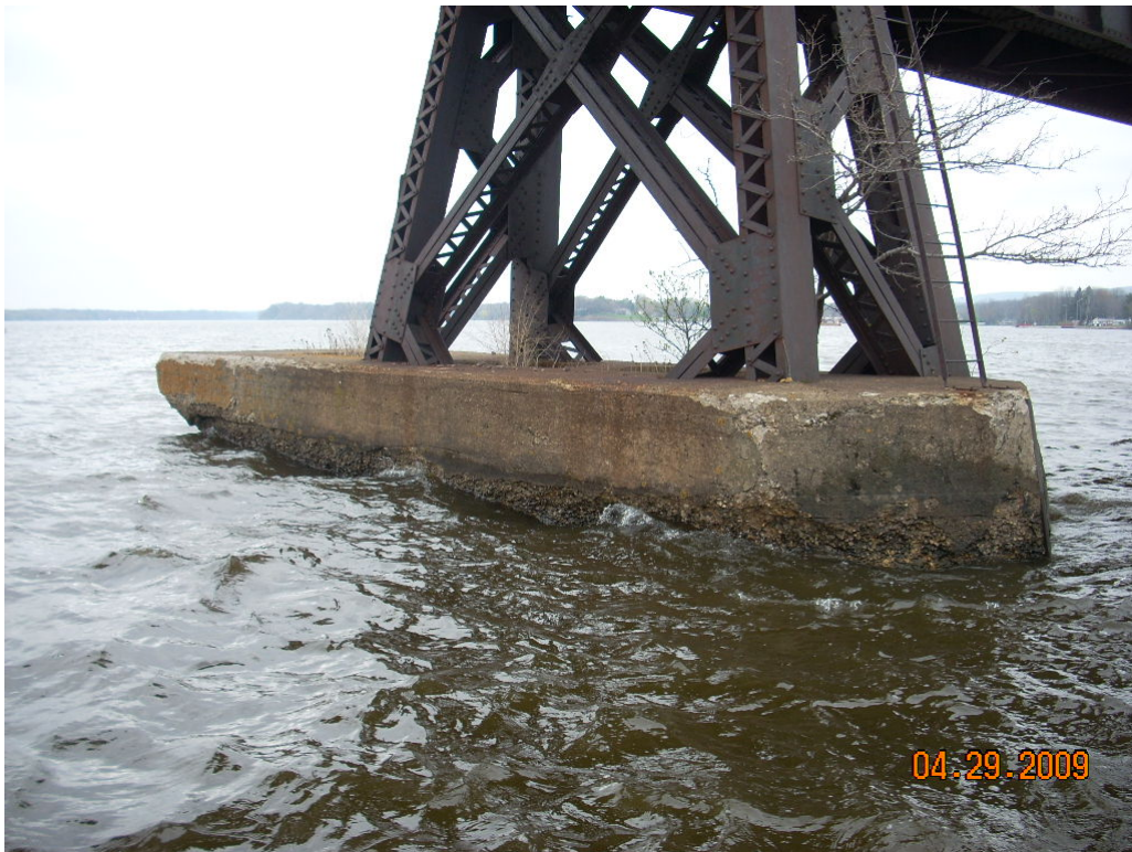
East Side of Pier 14
