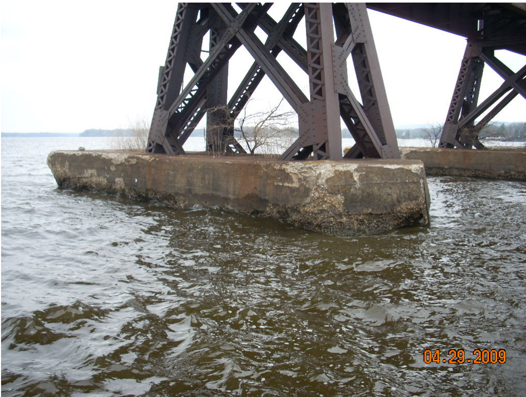
East Side of Pier 8
