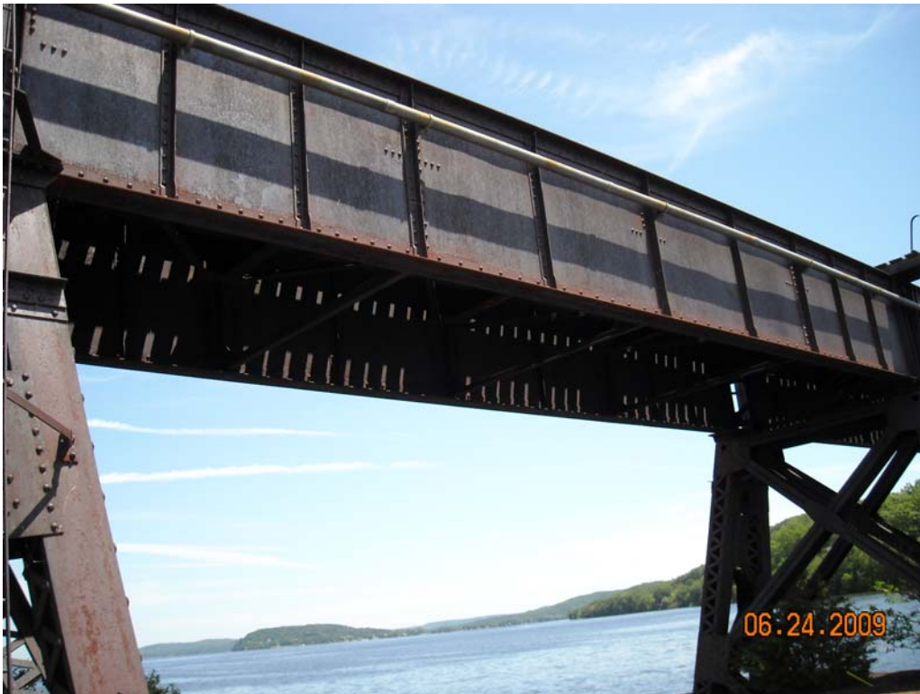
Typical Downstream (South) Profile of Deck Girder Span
