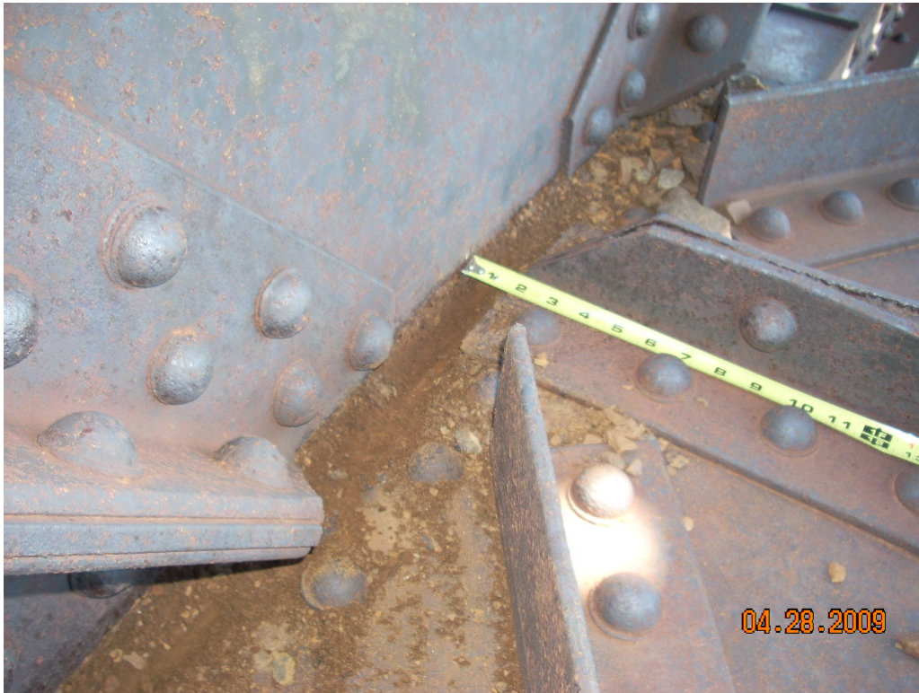
Typical pitting up to 25 percent of thickness of vertical gusset plate at lower chord connections where rock and soil are present
