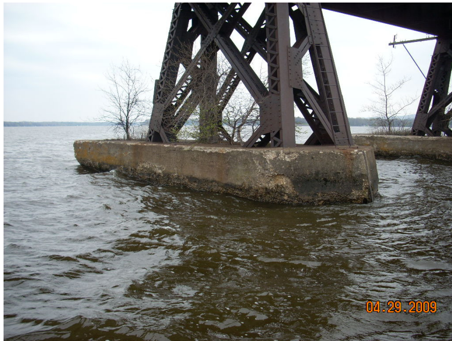
Figure 2-6 Typical View of Concrete Encased Tower Pier
