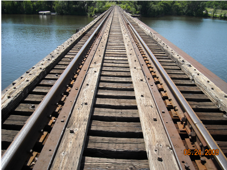
Figure 2-1 Typical View of Open Deck
