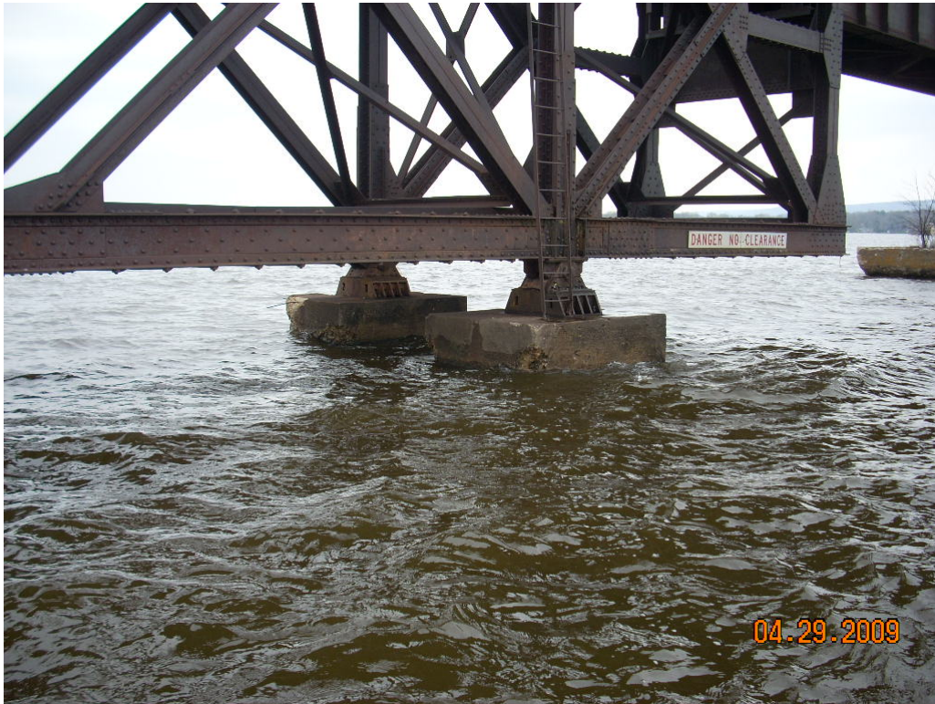
East Side of Pier 3
