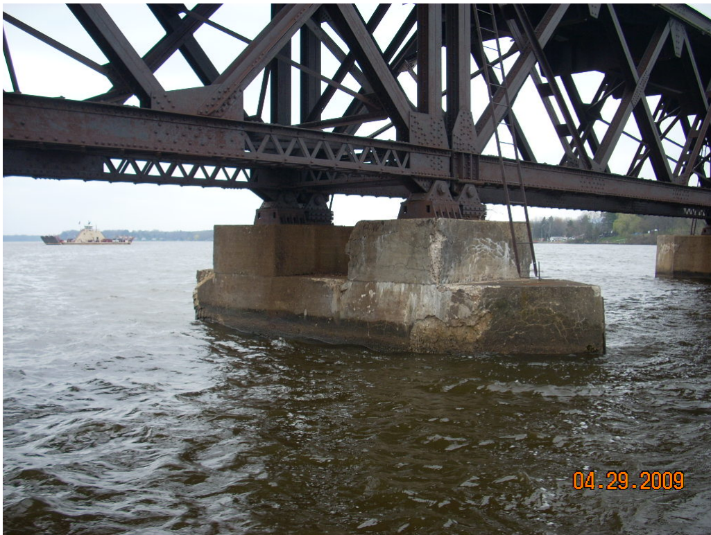
East Side of Pier 16
