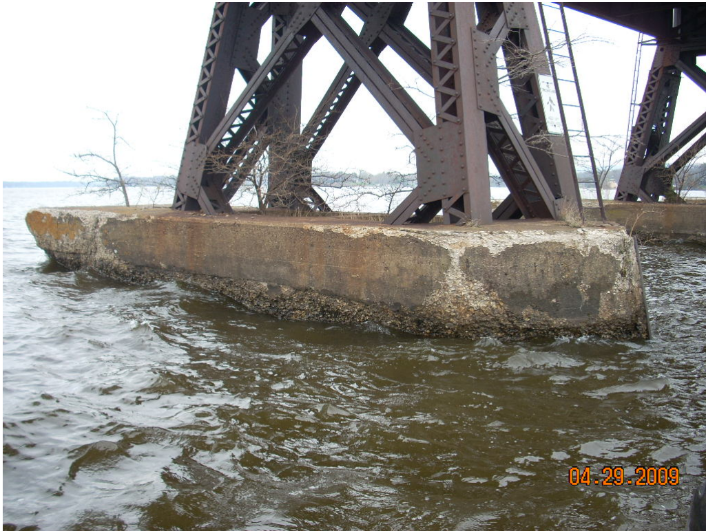
East Side of Pier 9
