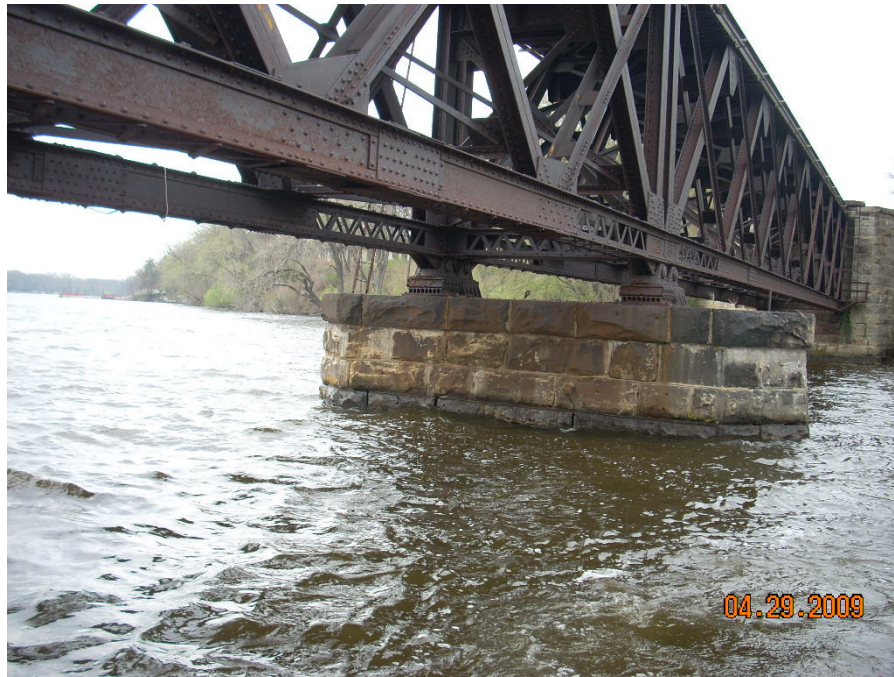
Figure 2-5 Pier 22, Typical View of Masonry Piers
