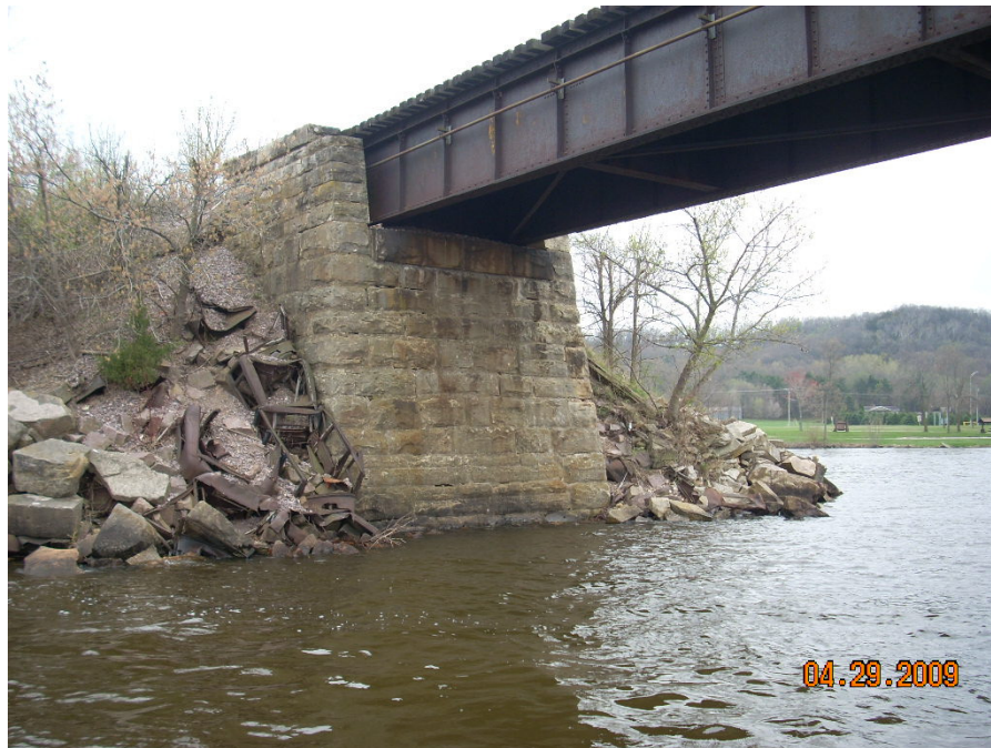
Figure 2-4 View of Abutment 1
