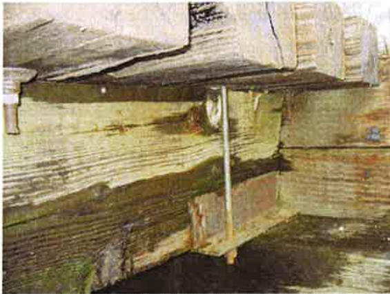
B-260 Splayed Cracking/Crushing Stringer 1, Span 1
