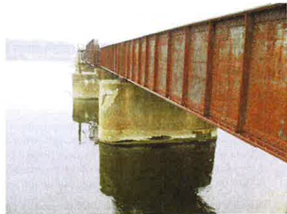
B-260 Concrete Shear Crack, & Concrete Erosion/ Pop outs at Cold Joint at Waterline Pier 2 -3/9/10 View West
