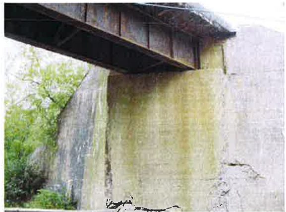
A-444 East Abutment Shear Cracks, Bearing Shaft & Bearings 1 & 2
