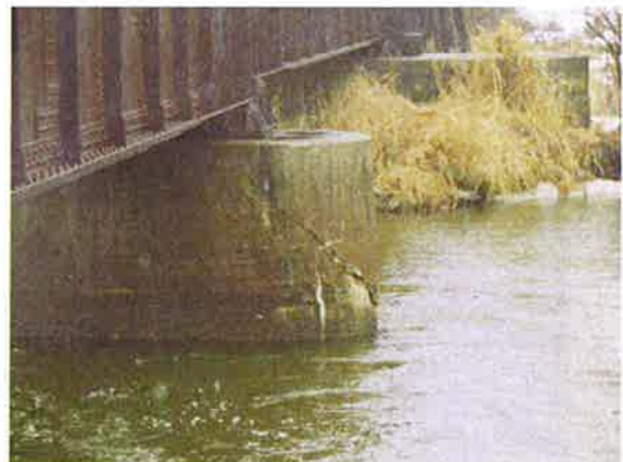
B-310 Concrete Shear Crack, Pier 2 -3/11/10 View East
