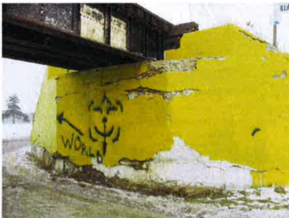
A-454 East Abutment Shear Cracks, Bearing Embedment January 2010
