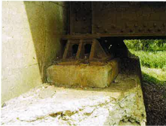
A-440 Concrete Conditions East Abutment Bearing 2
