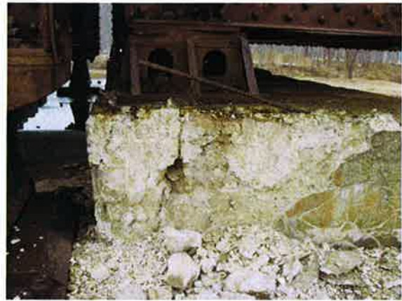
B-260 Shear Fractured Concrete -25% of Load Bearing Area, Bearing 5 Riser, North Face, Pier 3, Span 8 -3/9/10
