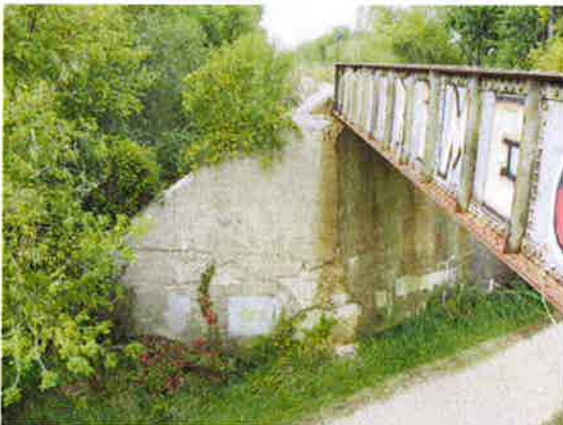
A-446 West Abutment Shear Cracks, Under Bearings and Bearing Shaft
