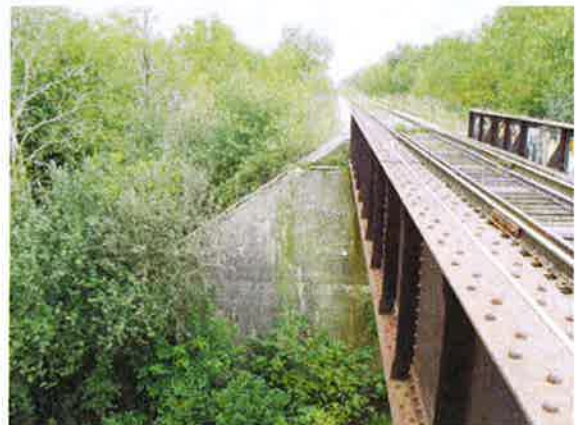
A-446 East Abutment Shear Cracks, Bearing Shaft & North East Wingwall
