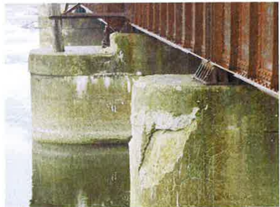
B-260 Concrete Shear Crack, Pier 2 -3/9/10 View West
