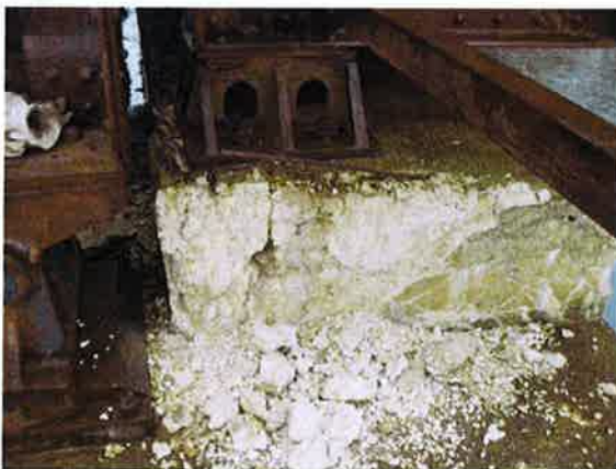
Fracture Detail Depth Bearing 5 Riser, North Face, Pier 3 -3/9/10
