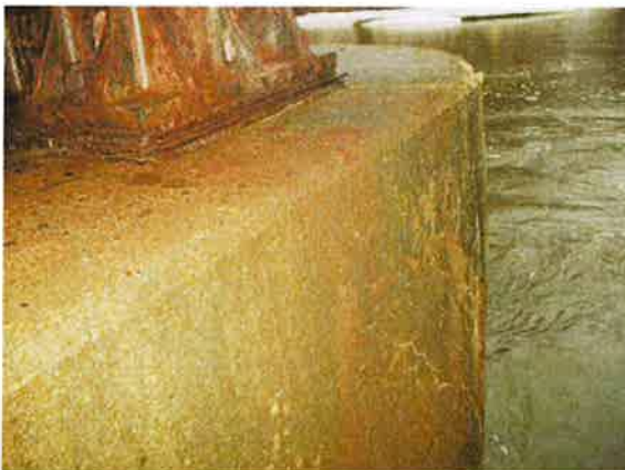
B-310 Concrete Bulging Shear Crack, Pier 2 -3/11/10 View South
