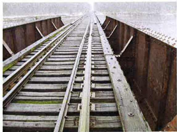
B-260 Tie Deck Span s 14 & 15 March 2010 View East (Note 12 Consecutive Ties Missing Spikes in Foreground)
