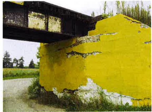
A-454 West Abutment Shear Cracks, Bearing Shaft November 2009
