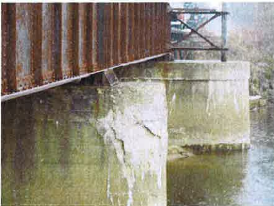
B-260 Concrete Shear Crack, Pier 2 -3/9/10 View East
