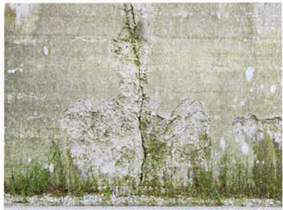
A-444 Vertical Column Cracks, Bearing Shaft & North West Wingwall
