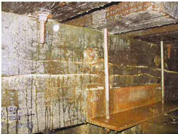
B-318 Bent 2, Span 1 & 2 Splayed Cracking/Crushing Stringer 1
