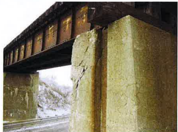
A-458 Pier 1 Shear Crack, Bearing 1 January 2010
