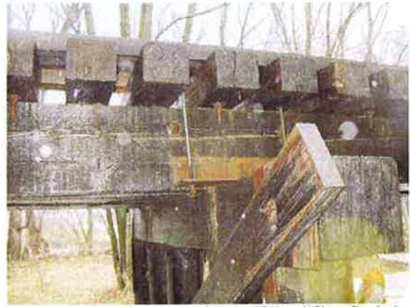
B-318 Bent 6 Pile Cap Fracture Stringer 1 Splayed/ Shear Cracked
