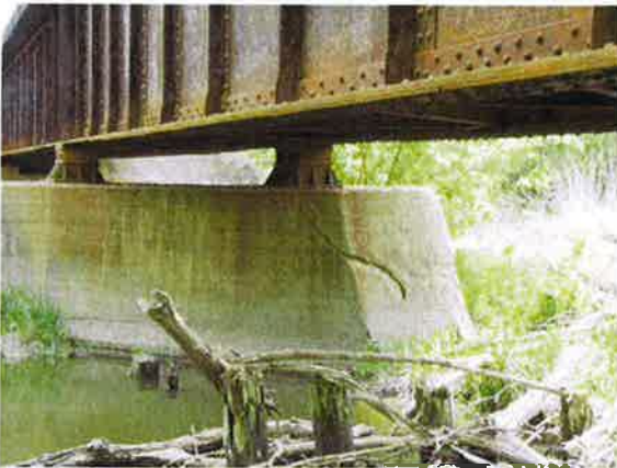
A-440 Concrete Shear Crack Under and Past Bearing 1, Pier 1
