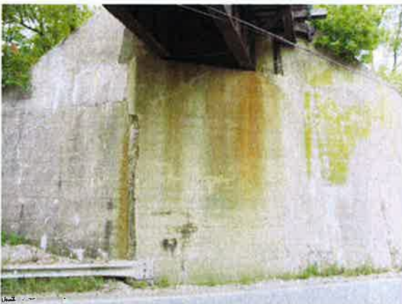
A-444 West Abutment Shear Cracks, Under Bearings 1 & 2 and Bearing Shaft
