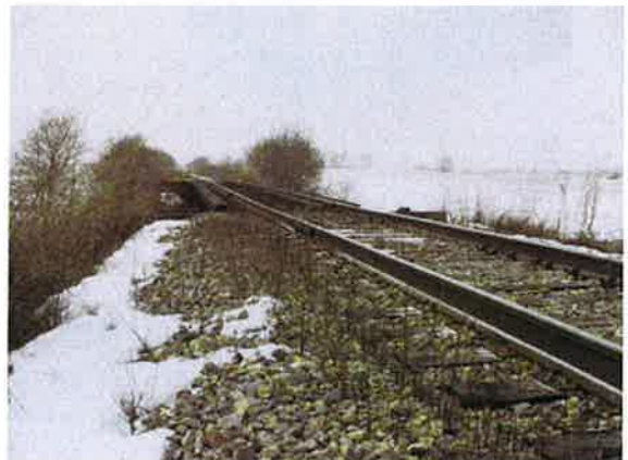
A-458 Typical Timber Trestle Approach Settlement January 2010
