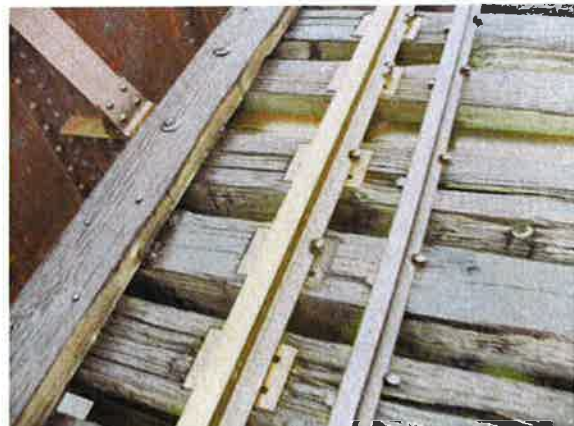
B-260 Typical Tie Deck Condition Spans 14 & 15 March 2010
