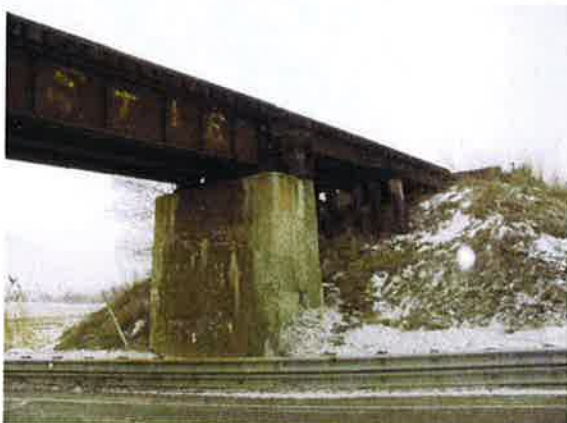
A-458 Pier 2 Shear Cracks around Pier Periphery January 2010
