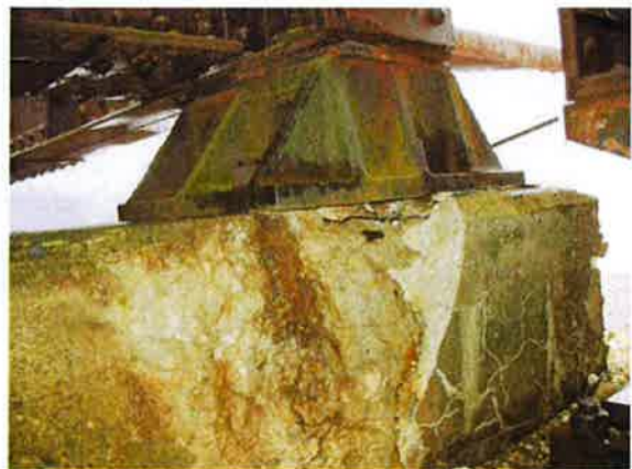
Fractured/Displaced Concrete Load Bearing 5 Riser, West Face, Pier 3 -3/9/10
