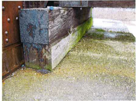
B-260 Sub Cap(lower) Frame Bent 6 Cracking/Crushing (pier 1)
