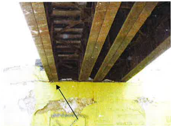
A-454 West Abutment Stringer Beam 1 Rotation/Embedment January 2010
