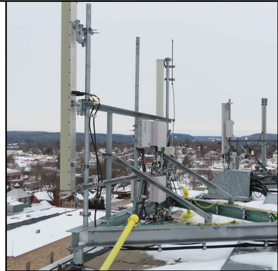
B EXISTING (ALPHA SECTOR) ANTENNA PLATFORM
