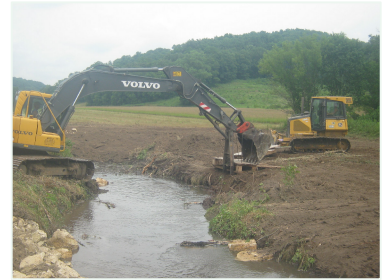
CONTRACTOR INSTALLING LUNKER
