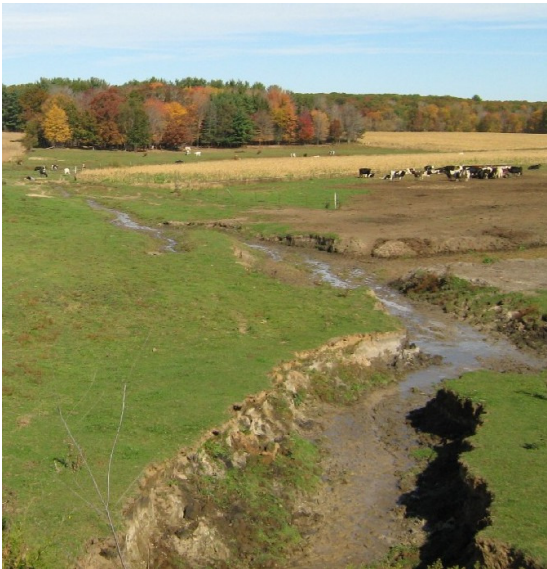
Large gully site undermining a county highway, fall 2008
