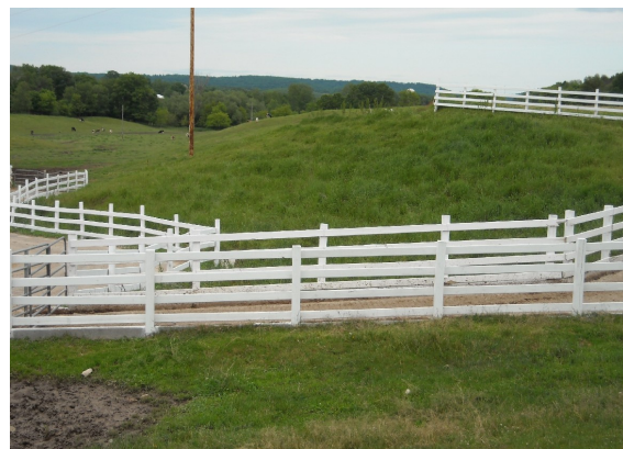
Same site in 2009, looking east
