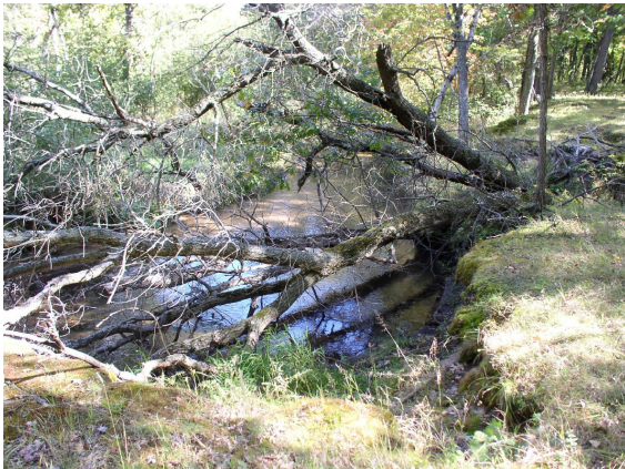
Eroded Lyndon Creek bank before construction
