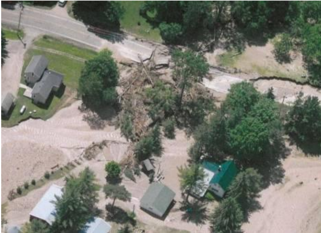
Figure 3: Aerial Photograph of Debris Jam at STH 113 Culvert #1
