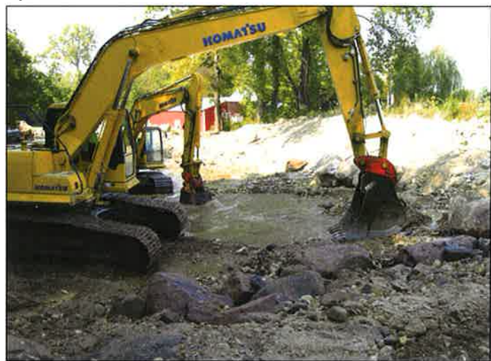
Construction of desiltation basin in Clark Creek Channel.
