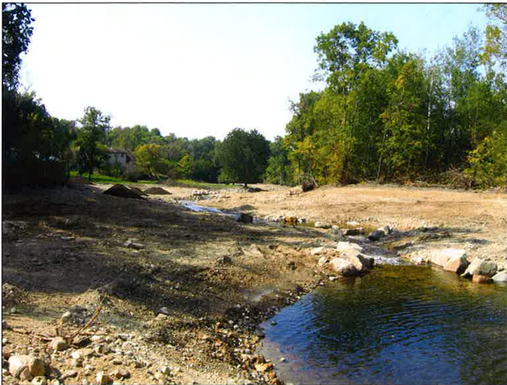
Desiltation basin at upstream extent of rechannelization of Clark Creek.
