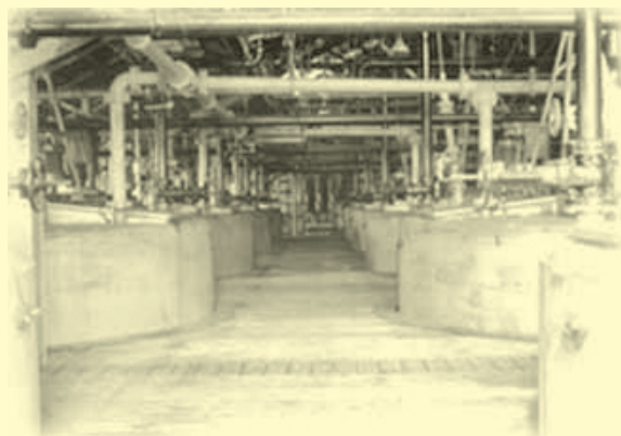
Stainless Steel Holding Tanks- Photo from UW-Madison's CAE Website: homepages.cae.wisc.edu/.../nov00/ammunition.html
