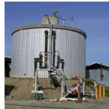
Manure digesters allow farmers to turn manure into profit by creating renewable energy.
