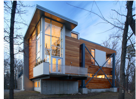
Reusing materials lowers the environmental impact of housing. This house was made using parts of an interstate that was rebuilt.
