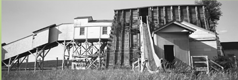
An escape chute from a structure at BAAP. Source: Jill Metcoff Photography
